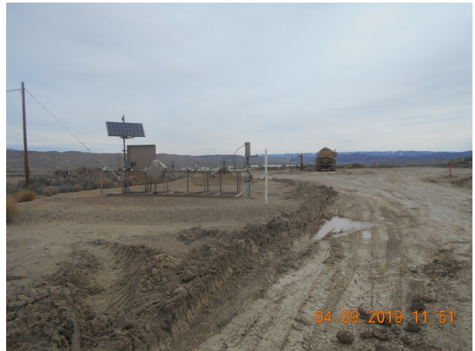
Injection wellhead and WAG Skid
