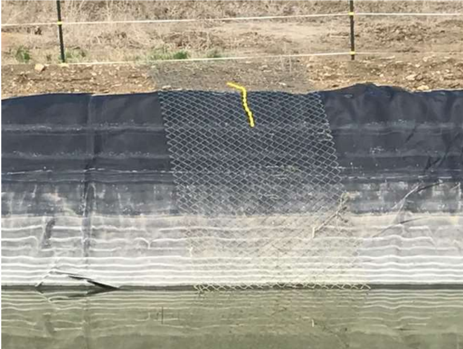
PHOTO 5: A YELLOW CHAIN WAS INSTALLED ON THE PRODUCTION PIT WALL INDICATING TWO FOOT OF FREEBOARD BETWEEN THE TOP OF THE PIT WALL AT ITS POINT OF LOWEST ELEVATION AND THE FLUID LEVEL.
