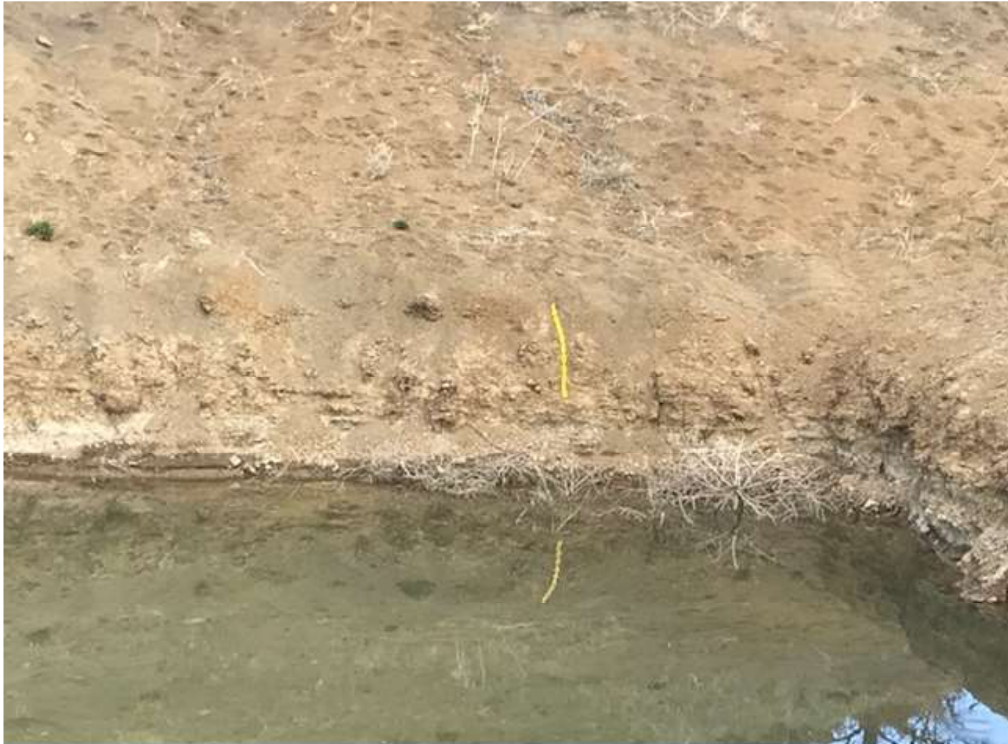
PHOTO 3: A YELLOW CHAIN WAS INSTALLED ON THE PRODUCTION PIT WALL INDICATING TWO FOOT OF FREEBOARD BETWEEN THE TOP OF THE PIT WALL AT ITS POINT OF LOWEST ELEVATION AND THE FLUID LEVEL.
