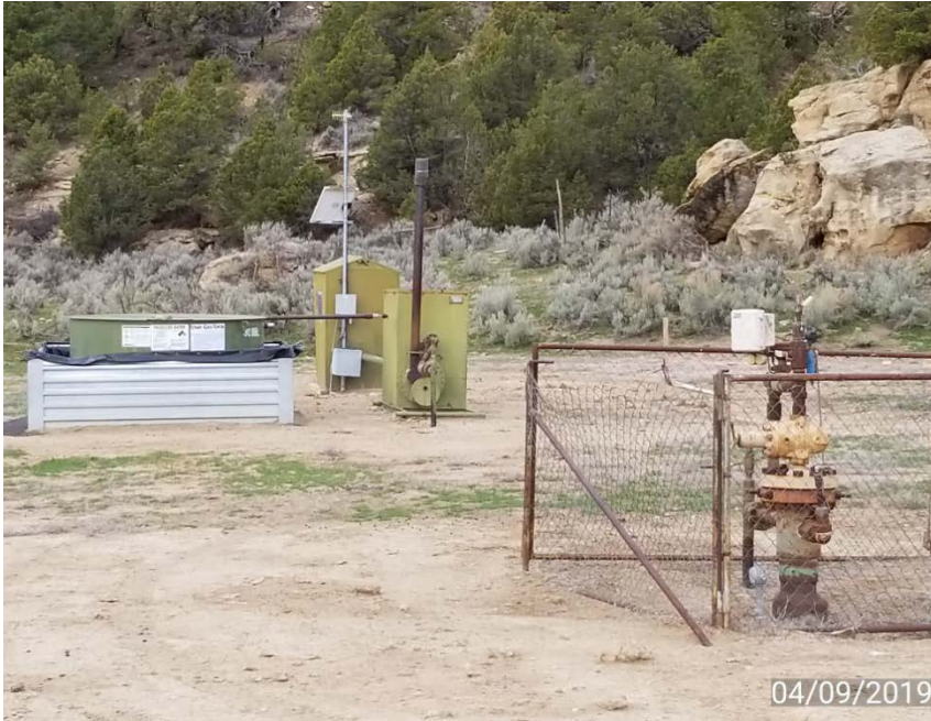
Photo 1. Location looking southwest.
