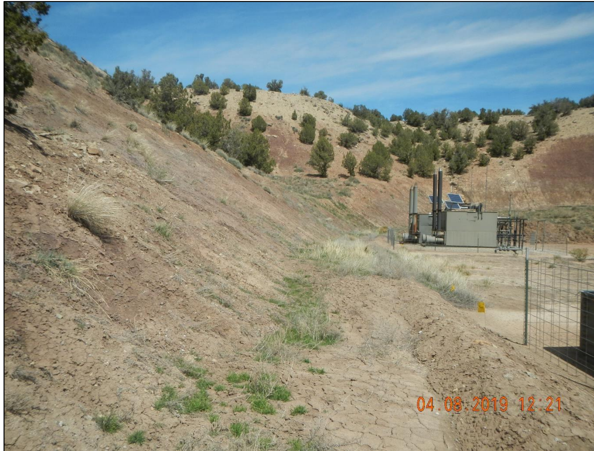
Sediment build up in ditch around cut slope.
