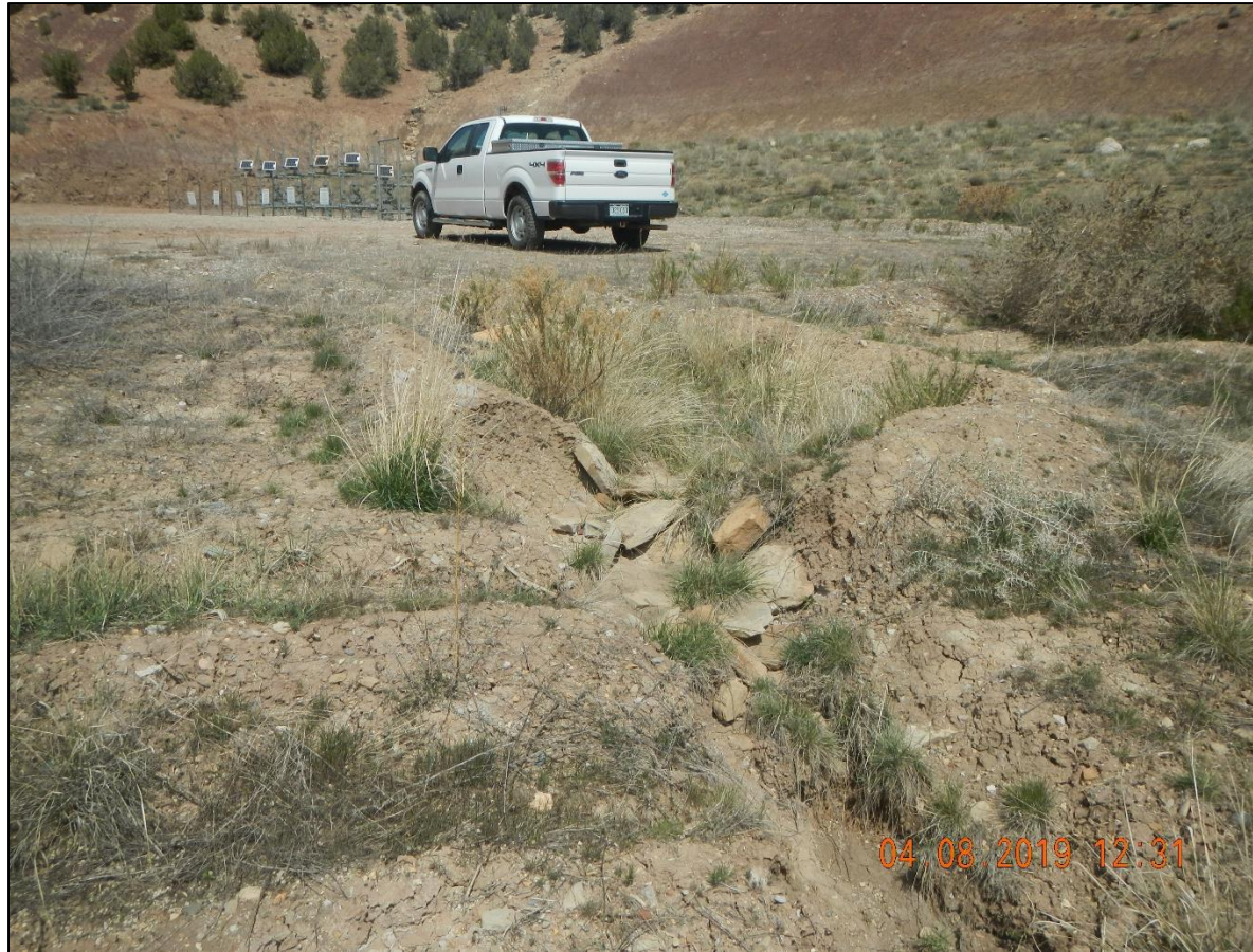
Checkdam is washed out and needs maintained.
