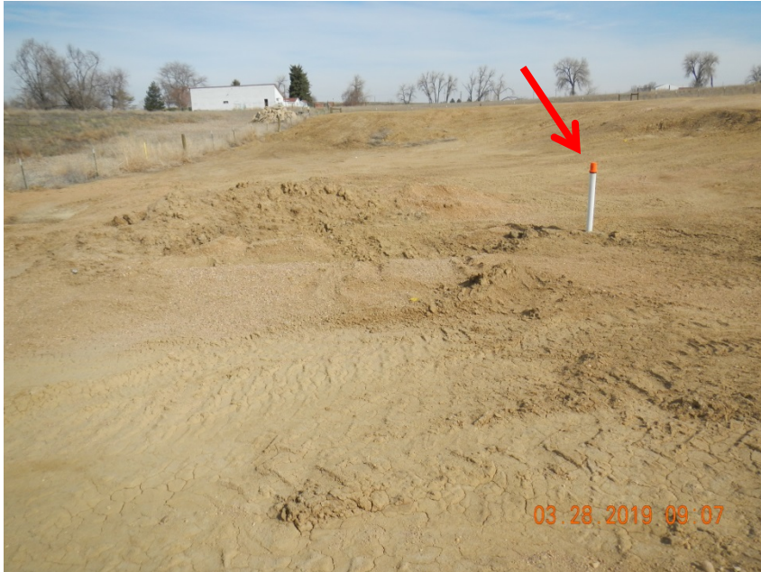
Photo 3. Photo taken from the location, facing Northeast. Photo depicts the removal of most equipment has been performed. However, equipment still remains on location. Gravel remains and location has not been re- contoured/re-graded.
