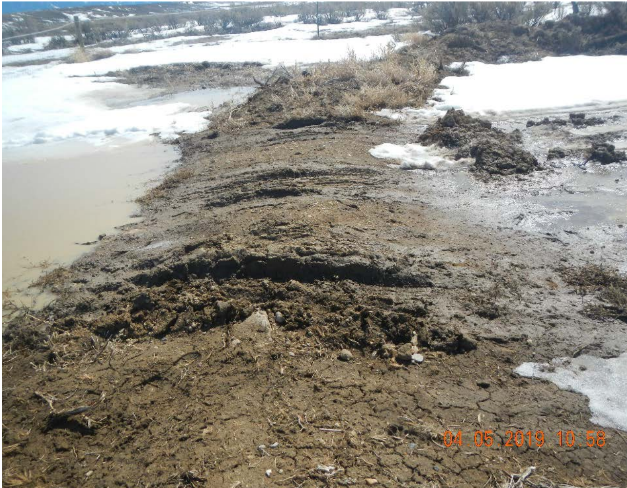
Photo 16 Drive over secondary containment at access to land treatment location.
