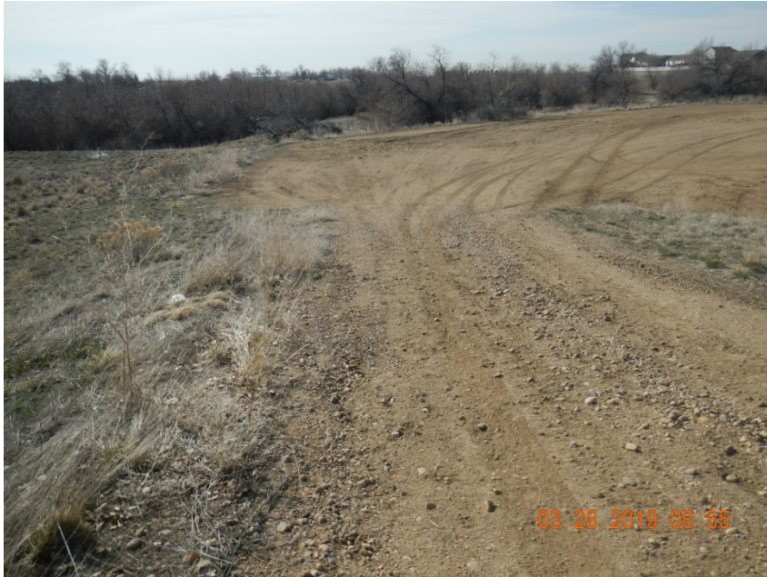
Photo 3. Photo taken from the access road looking into the location, facing Southeast. Photo depicts the removal of all equipment has been performed. However final reclamation activities have not been performed at the time of inspection.
