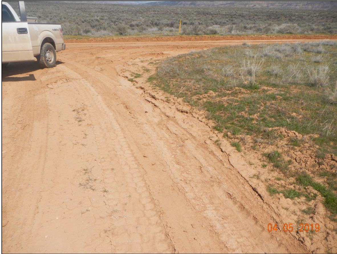
Photo #4 Erosion moving sediment off location at entrance with no BMP in place.
