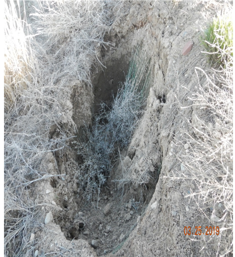
Photo#8: Point where stormwater discharges on outside of East Fill slope.
