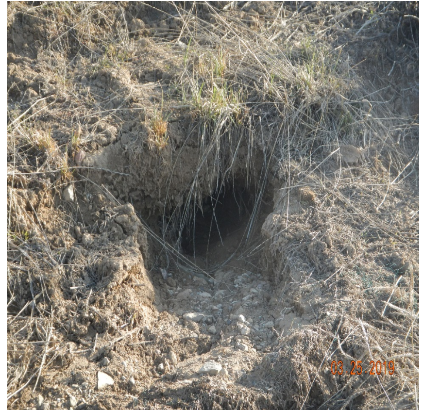
Photo#4: Point where stormwater discharges on outside of NW Fill slope.
