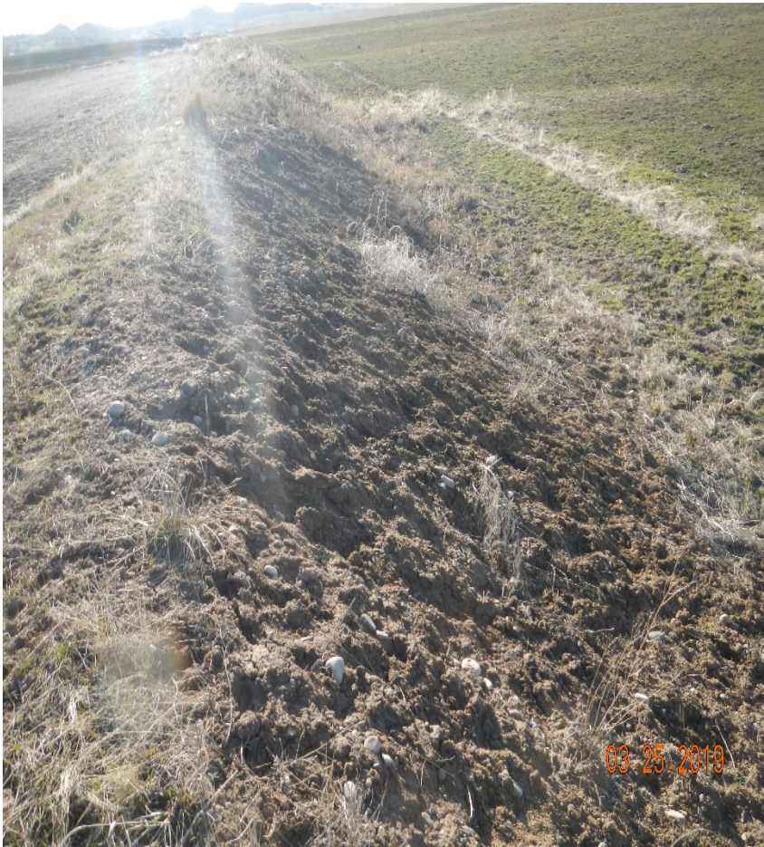
Photo#5: View over fill slope to West. Areas of fill slopes are in need of stabilization.
