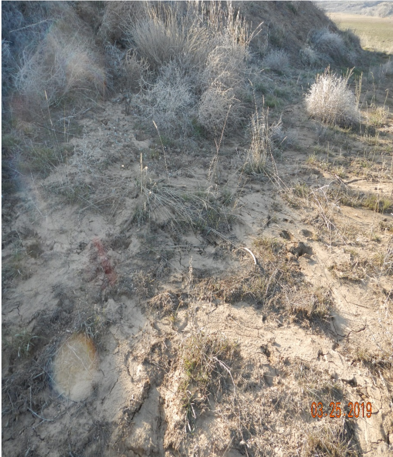
Photo#9: Base of East fill slope showing Sediment migration.
