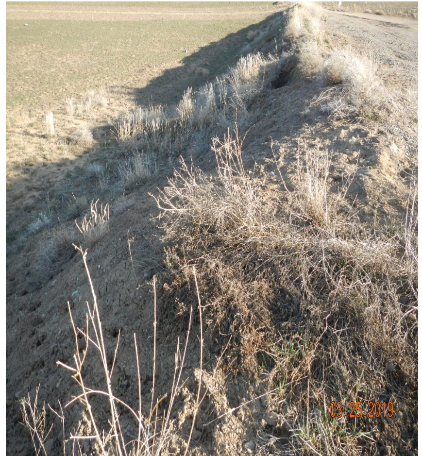
Photo#6: View over fill slope to East. Areas of fill slopes are in need of stabilization.
