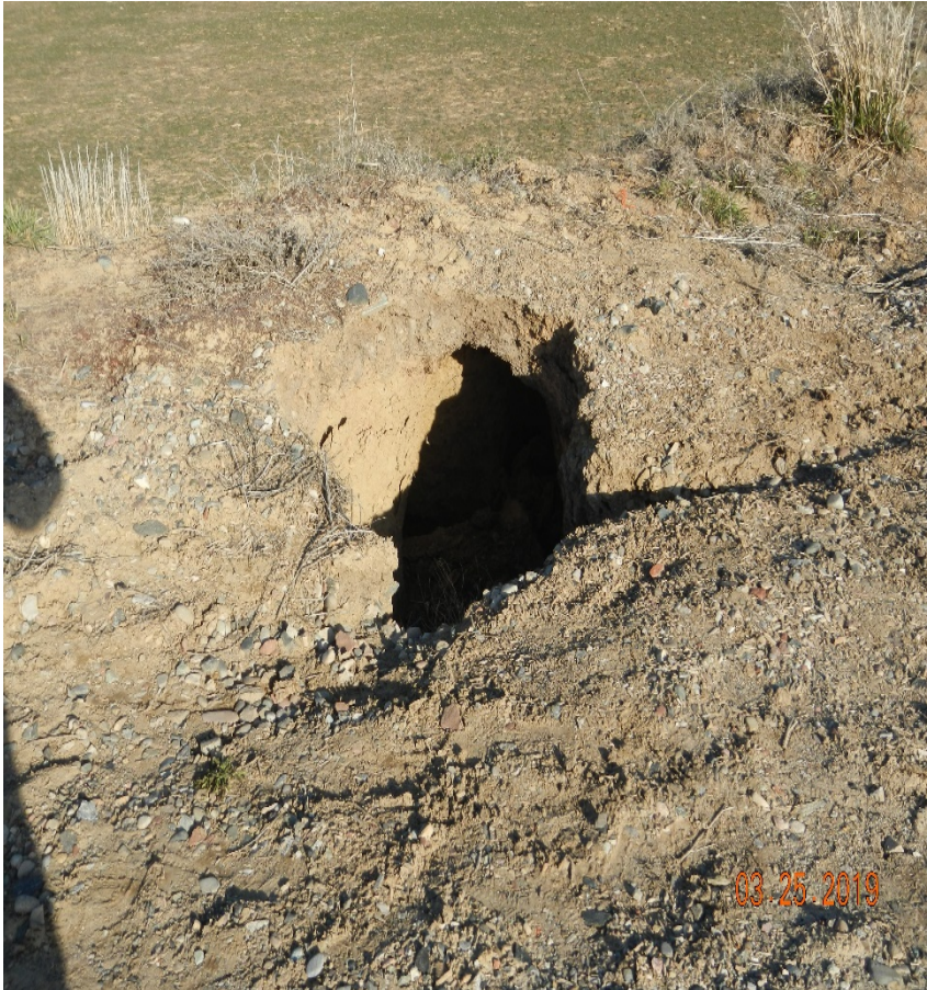
Photo#7: East side of Pad where Stormwater has collected & blown out channels through Fill slope.
