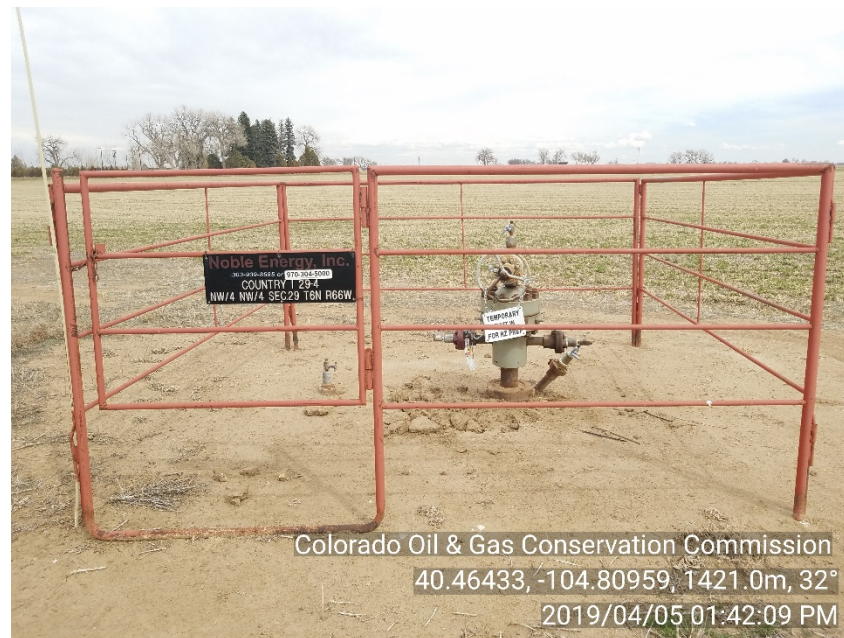
Photo #2 Country 1 29-4 Wellsite Temporarily Abandoned | TA Unused Equipment - Removed Orange Decommission tag remains NOT present
