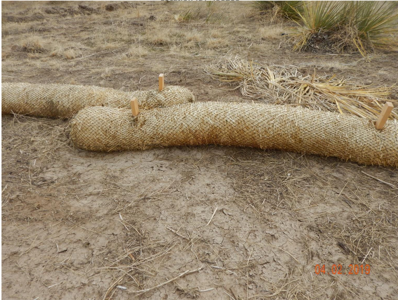
Photo 4: Photo taken from the east end of the location. Photo shows straw wattles have not been installed in accordance with good engineering practices.
