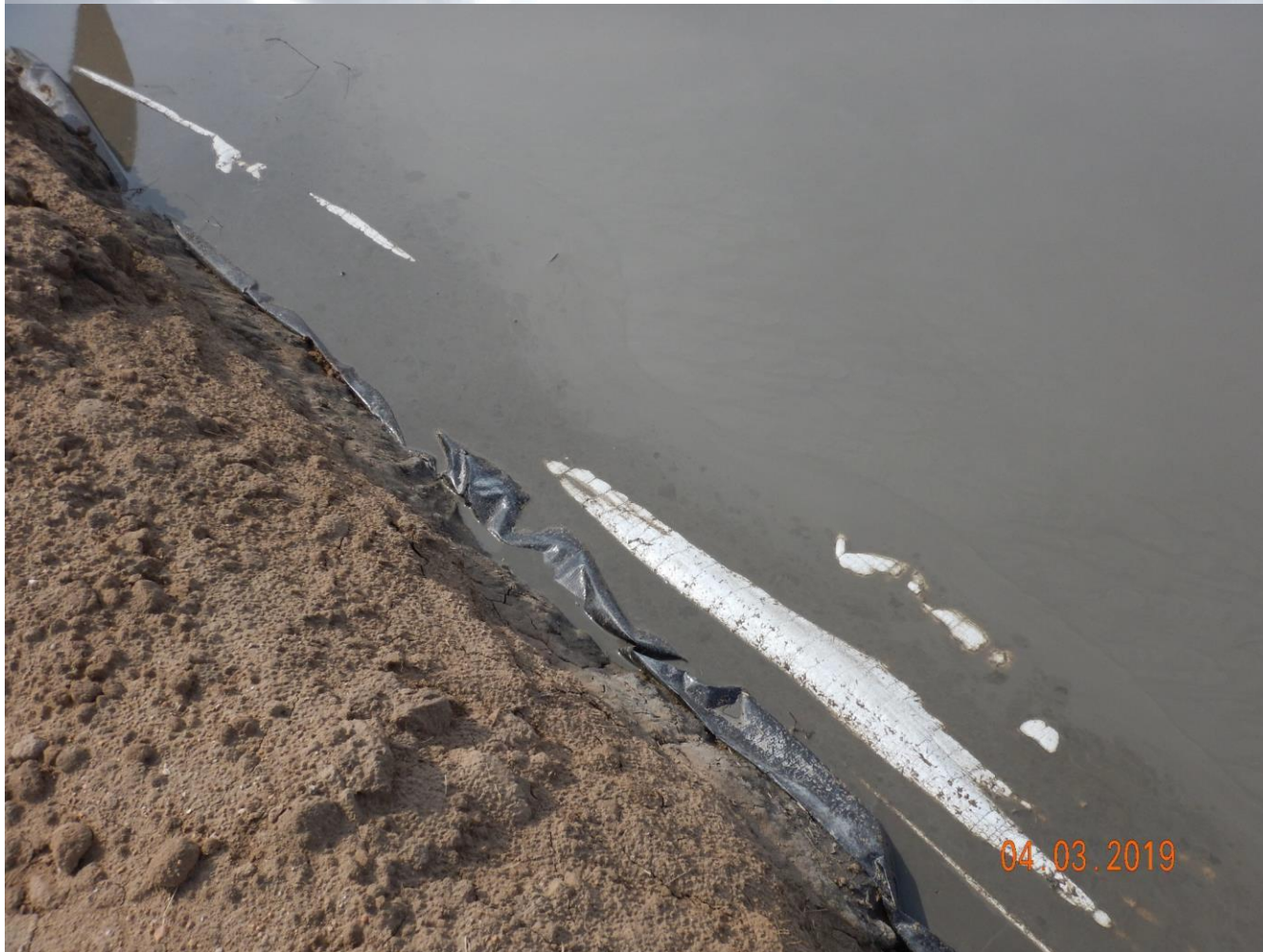
Photo 30: Photo taken from the drill pit. Photo shows section of the drill pit where the liner is no longer in proper functioning condition.
