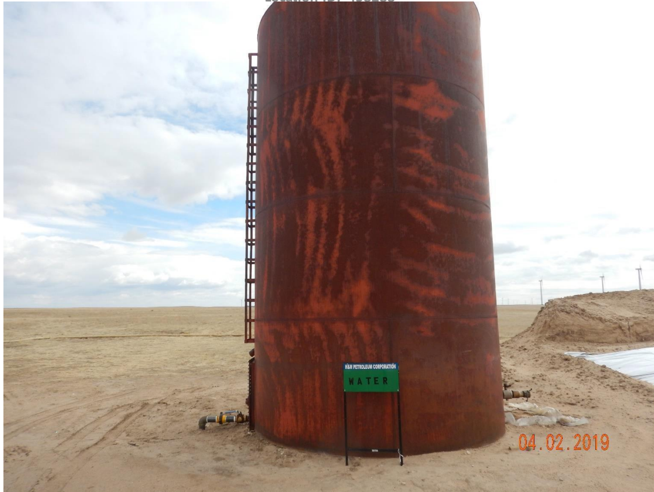
Photo 16: Photo taken from the produced water tank on the north end of the location. Photo shows insufficient signage (sign only says “water”) and labeling at tank in accordance with Rule 210.d. Photo also shows missing secondary containment at tank in accordance with 906.d(1).
