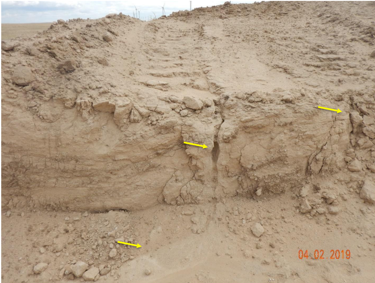
Photo 13: Photo taken from the soil stockpile. Photo erosion degradation due to stormwater
