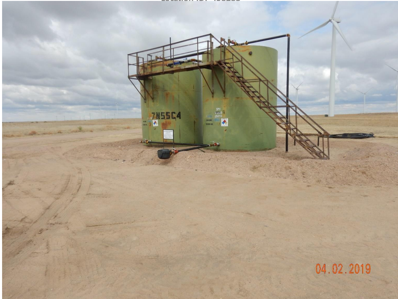
Photo 18: Photo taken from the north end of the location, facing northwest. Photo shows berm at battery appears to be unchanged. Operator does not appear to have installed secondary containment to comply with 906.d(1)
