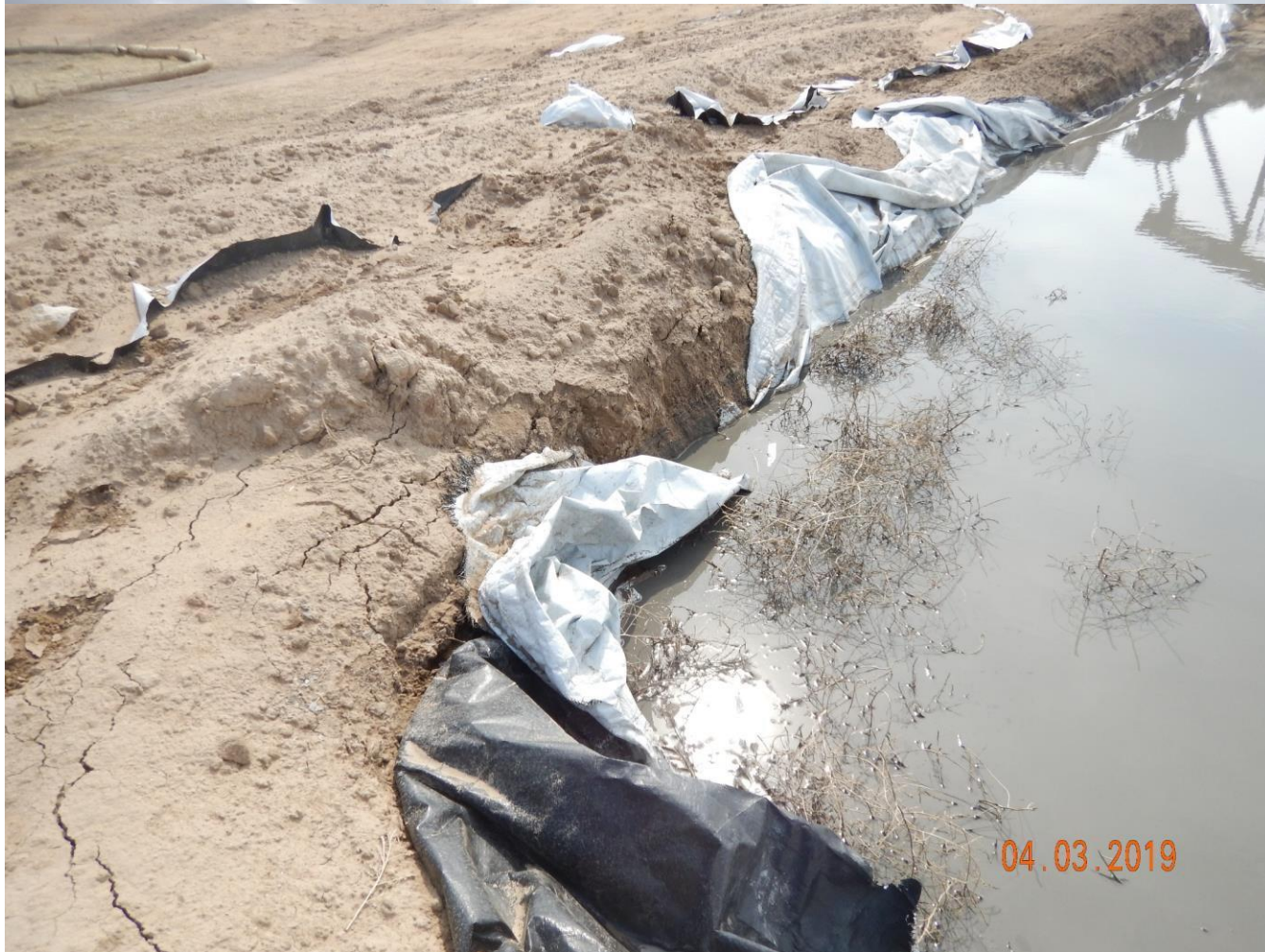
Photo 31: Photo taken from the drill pit. Photo shows section of the drill pit where the liner is no longer in proper functioning condition.
