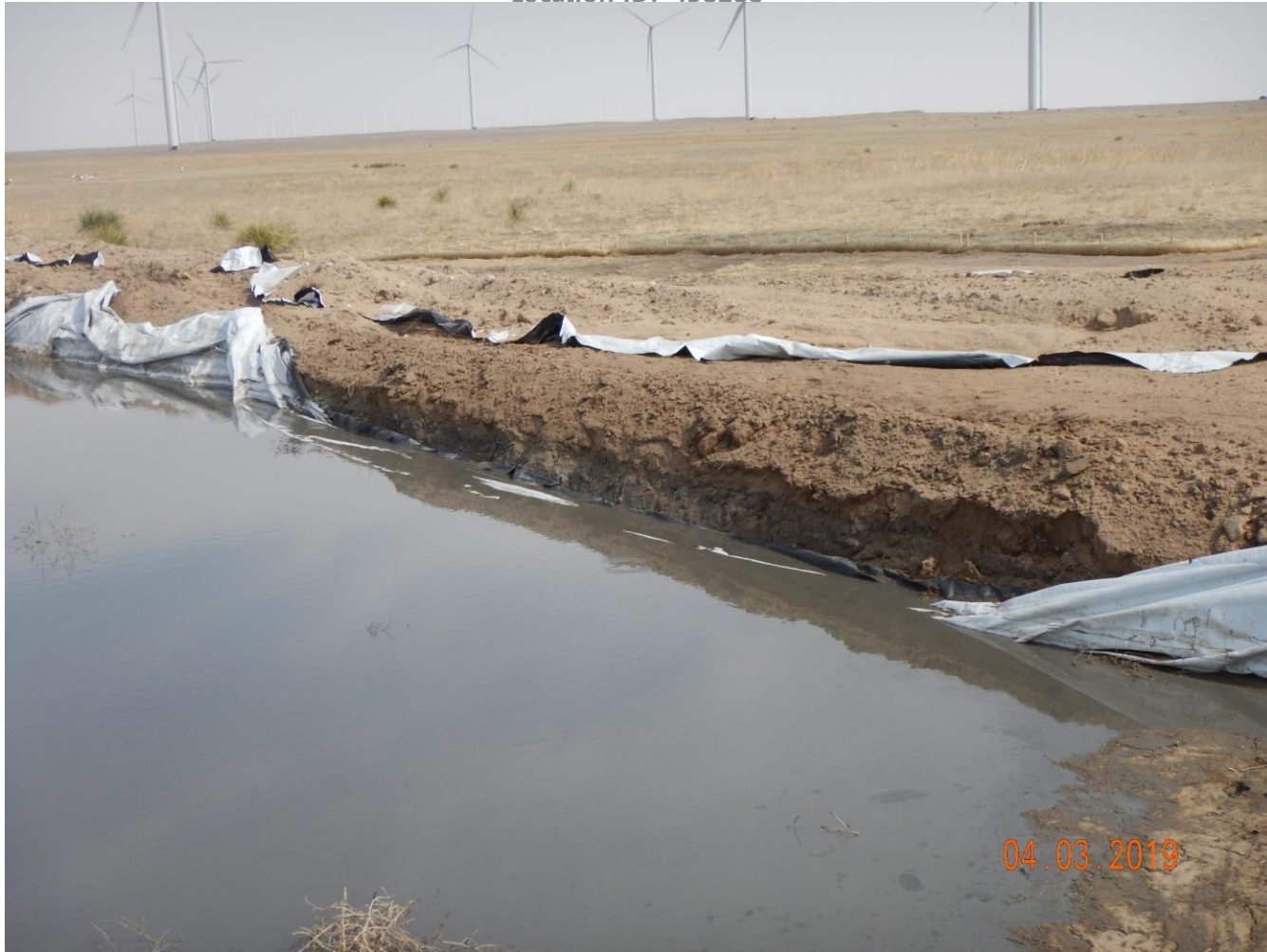
Photo 29: Photo taken from the drill pit, facing east. Photo shows section of the drill pit where the liner is no longer in proper functioning condition.
