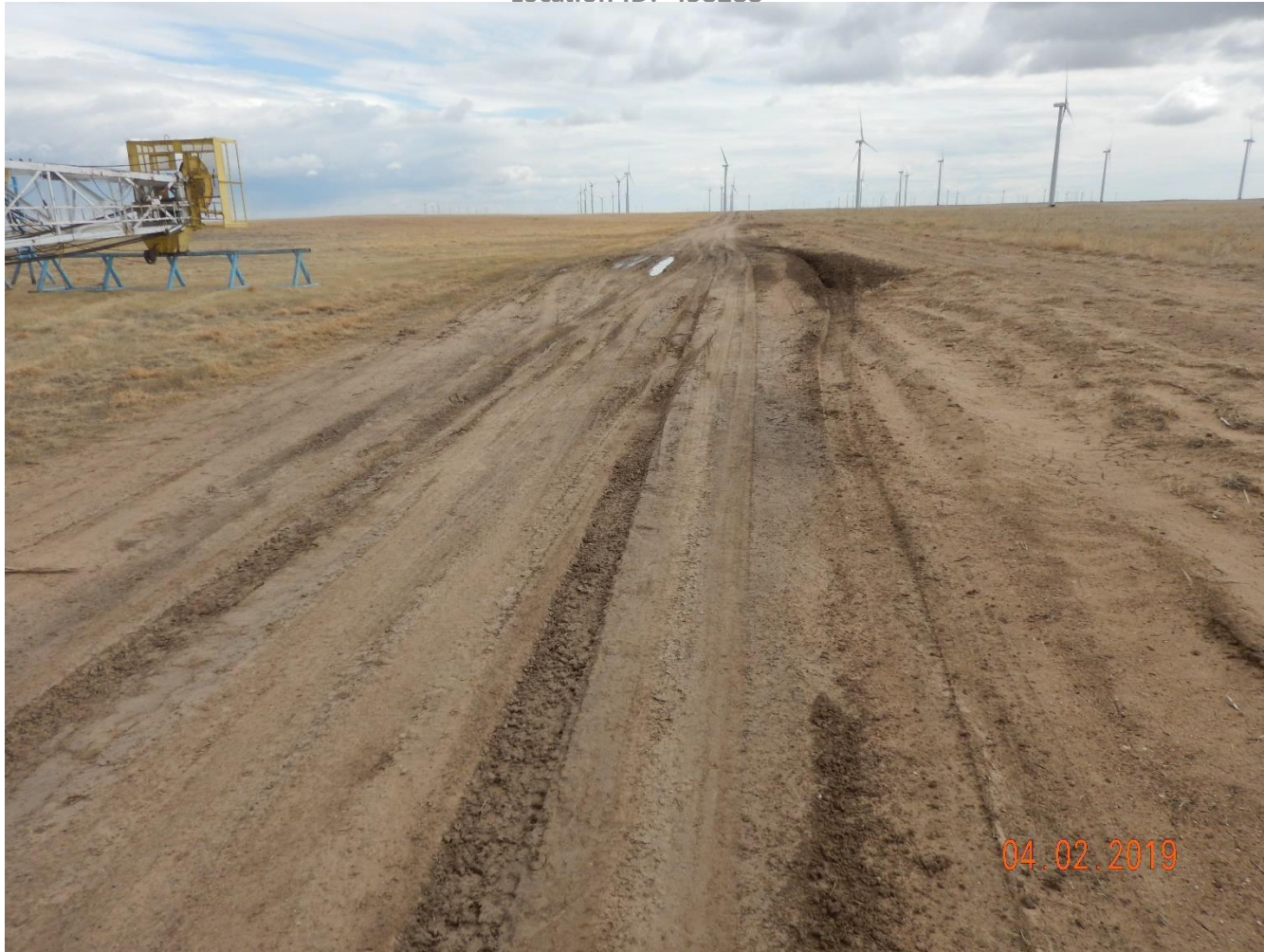
Photo 23: Photo taken from the from the east/west section of access road. Photo shows rutting degradation occurring along access road. BMPs should be installed and maintenance conducted to mitigate degradation to access road, and areas beyond the access road.
