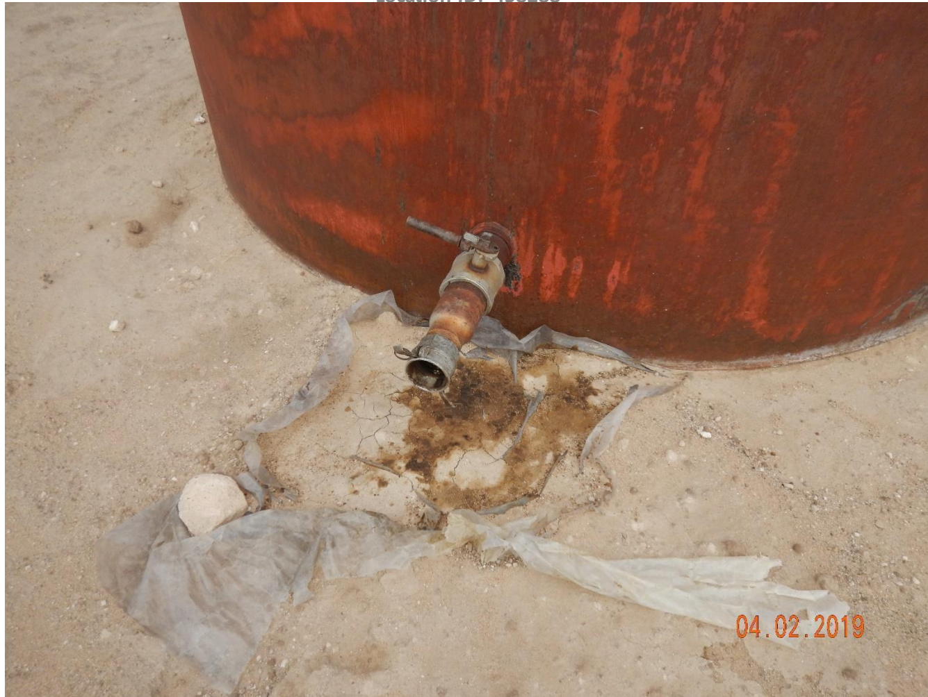
Photo 17: Photo taken from the south end of the produced water tank. Photo shows contaminated soils due to possible discharge from the tank.
