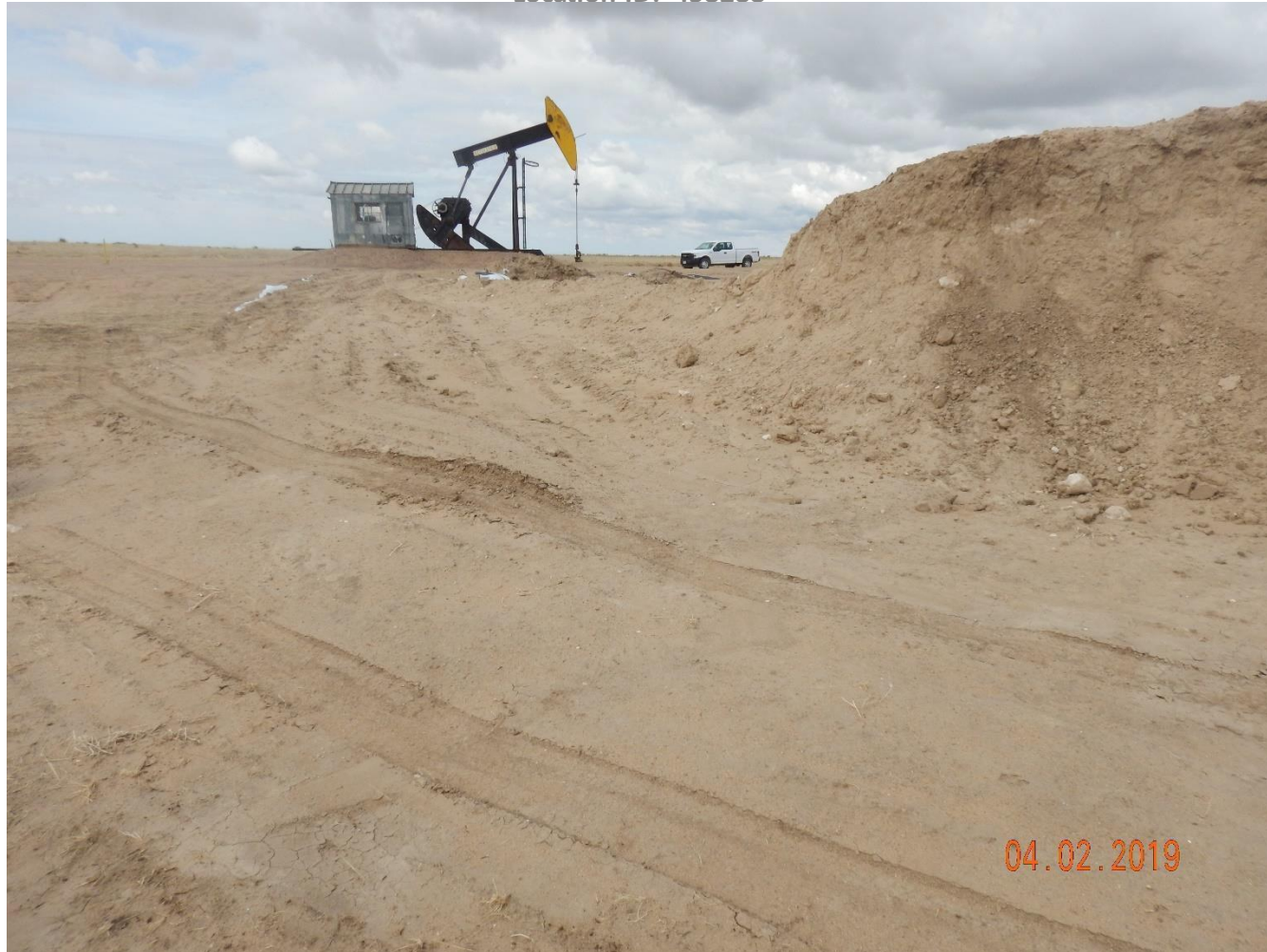
Photo 8: Photo taken from the east end of the location, facing west. Photos 8-10 provide overview from west, northwest to north, of the soil stockpile from pit. Photos show topsoil and the subsoil horizons were not separated and stored or marked/documentated in accordance with Rule 1002.b. Photos also show stockpile appears to remain loose, unstabilized material and stormwater erosion degradation is evident.
