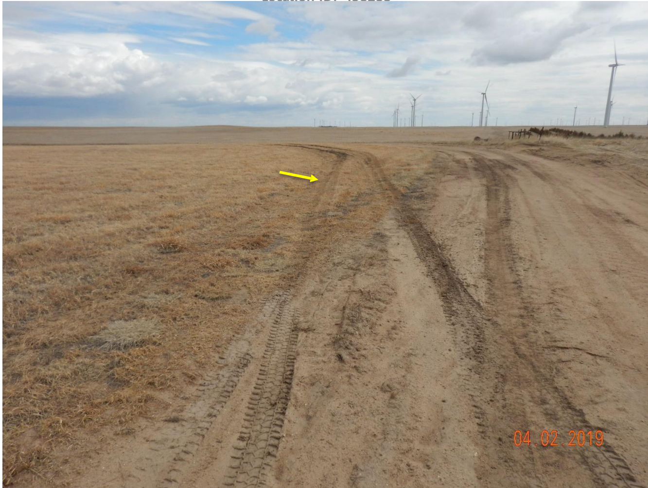
Photo 25: Photo taken northeast of the location, where the access road turns east/west to north/south. Photo shows operator appears to have travelled beyond the designated access road onto adjacent lands creating additional disturbance. This does not comply with 1002.e and will require reclamation.
