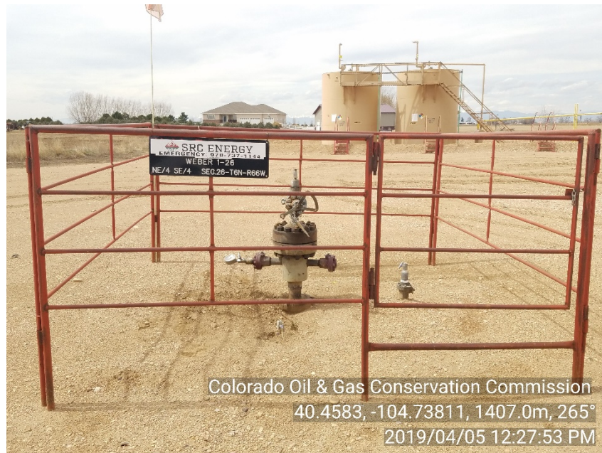
Photo #2 Weber 1-26 Wellsite Temporarily Abandoned | TA Unused Equipment - Removed
