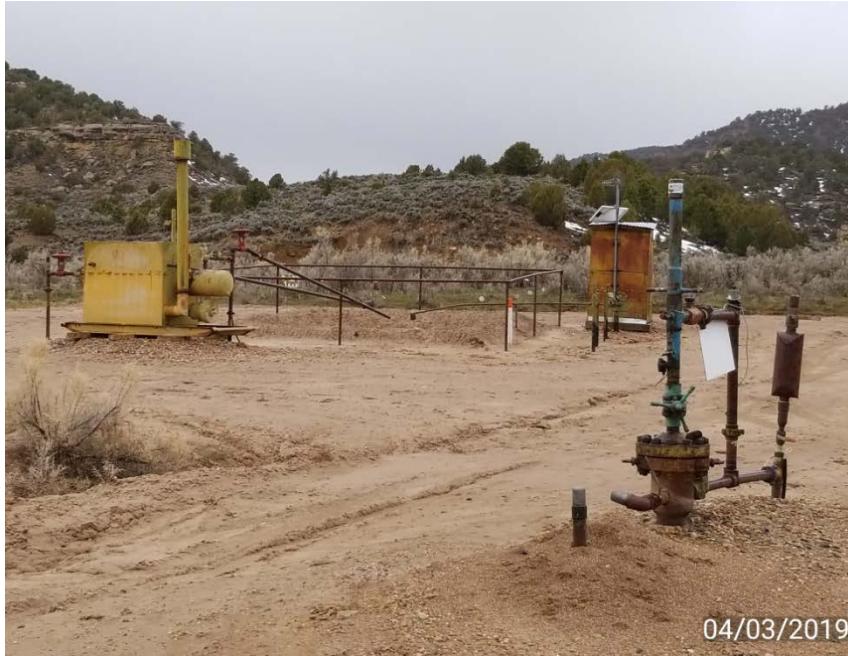
Photo 1. Location looking southwest.
