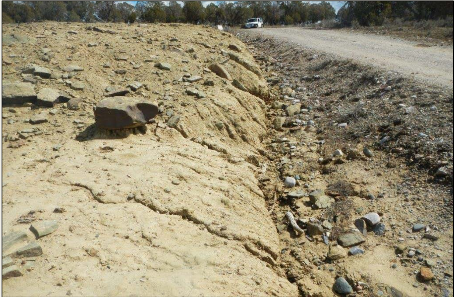
Photo 10. View of erosional channel approximately 3-4 feet wide and 3 feet deep, as well as erosional channels flowing into the channel, along the southern project area and access road.
