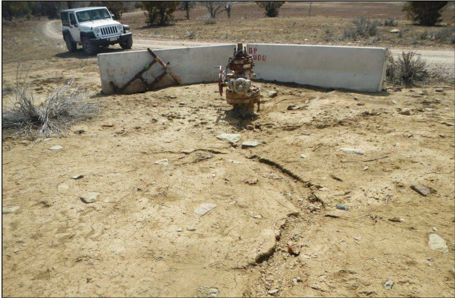
Photo 1. View of wellhead facing southward. Erosional channels is flowing around wellhead. Equipment placed next to jersey barrier does not appear to be functional and should be removed if not in use.
