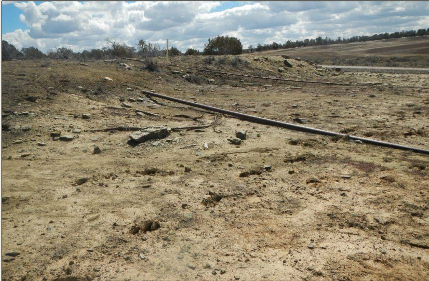
Photo 4. View of the western project area from the northwestern edge facing southward. Little desirable vegetation observed. Significant rilling from well pad fill slopes is occurring. Surface flow lines are not connected and decaying. These need to be removed.
