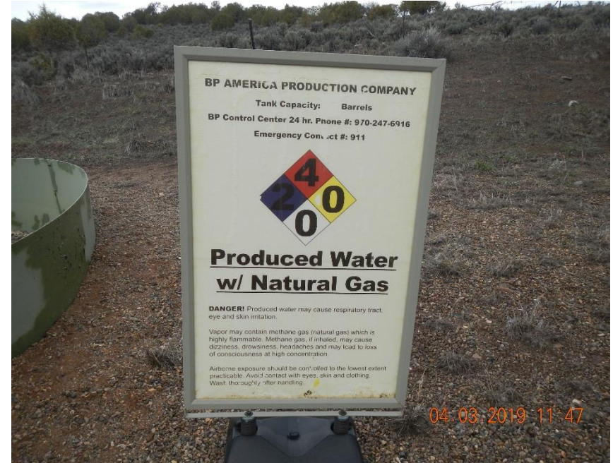
Capacity is not labeled on produced water sign.
