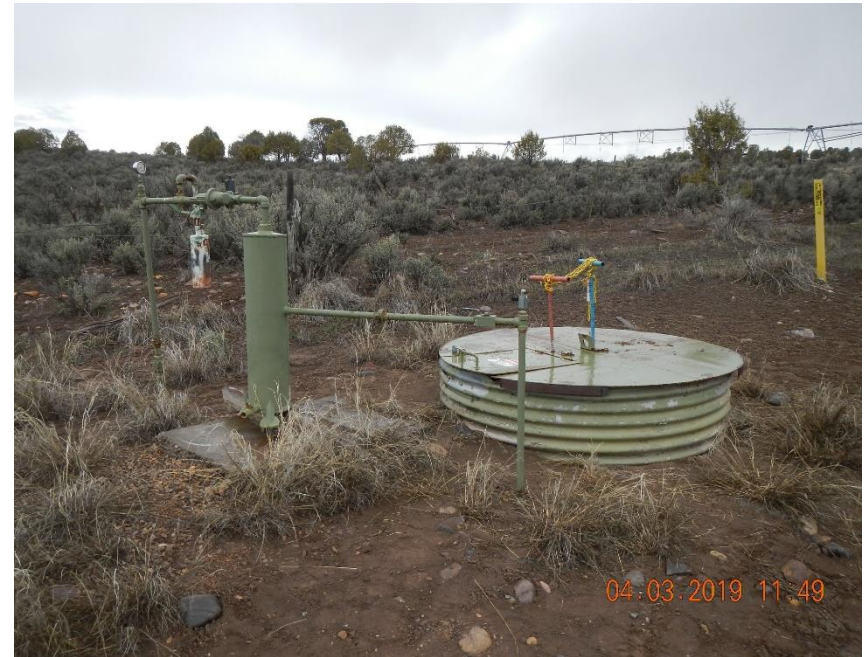
Domestic tap and valve can on western edge of location.
