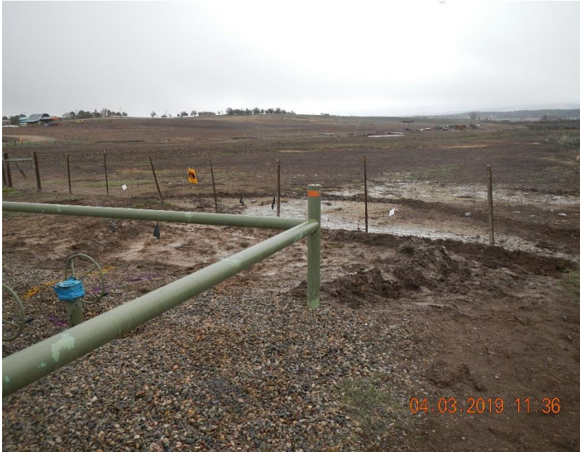
Dirt berms constructed in an attempt to contain fluids.
