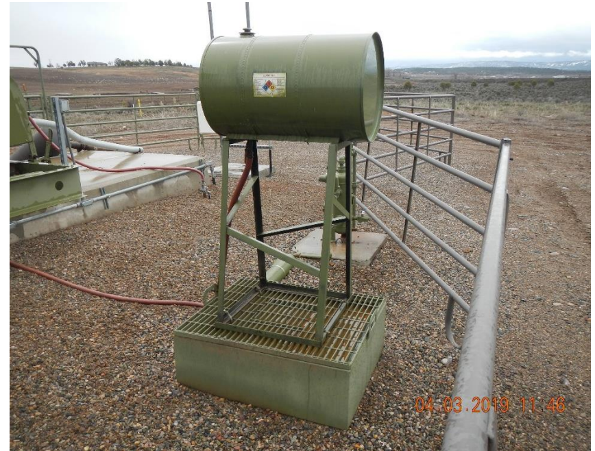
Lube oil container on secondary containment.
