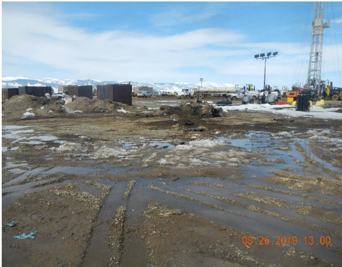
Photo 12- Overview of location taken at entrance facing east. Stained soil stockpiled were observed, soil should immediately be removed and handled per COGCC rule 907.
