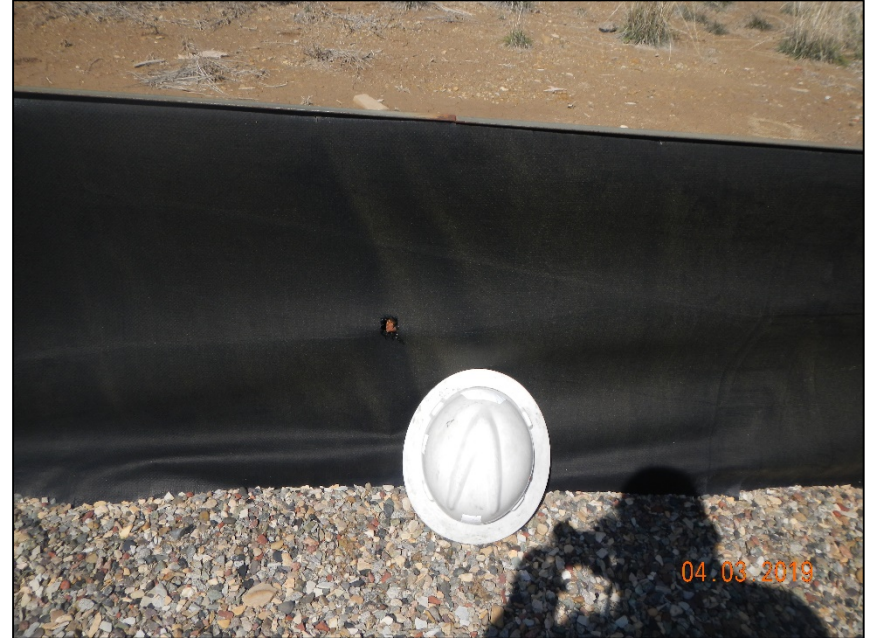
Photo # 6. Hole in liner inside of tank containment.
