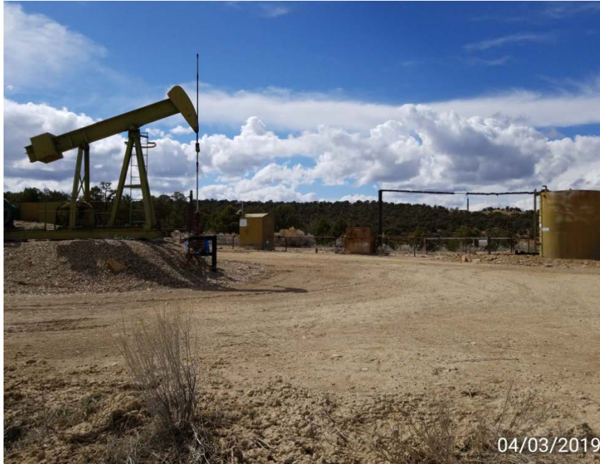
Photo 1. Location looking west.
