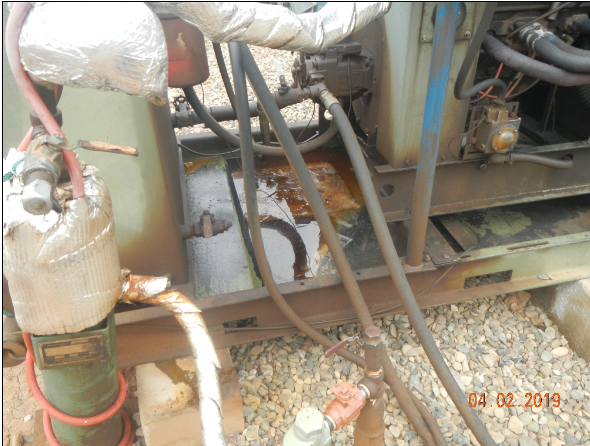
Photo 3. There is some oil on the engine skid.
