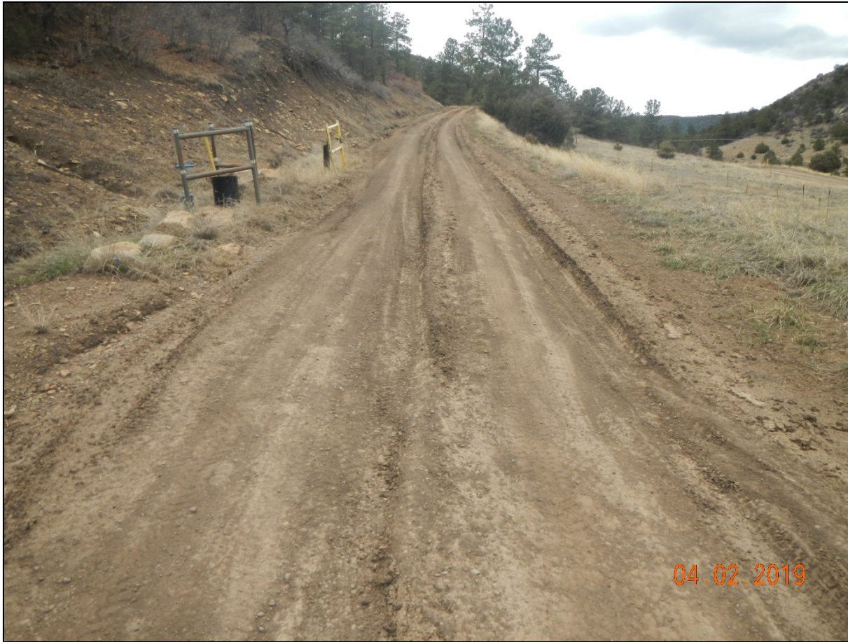
Photo 2. There is signs of erosion and vehicle rutting along the road that travels up to the location.
