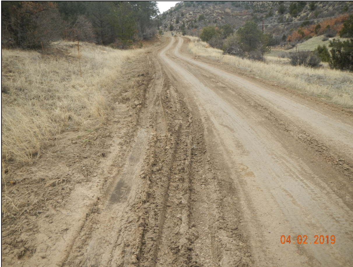
Photo 1. There is vehicle rutting along the main access road in the canyon.
