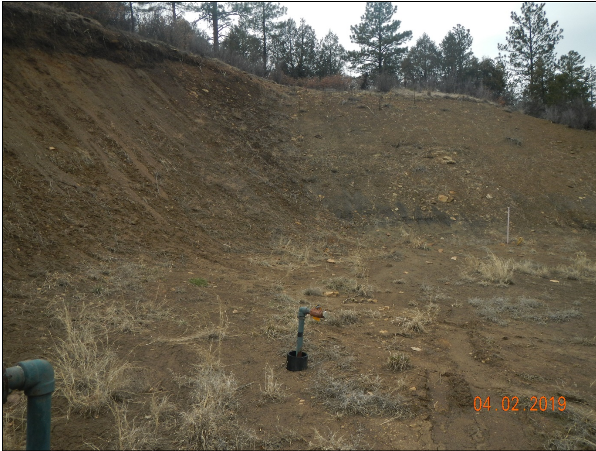
Photo 2. There is signs of sediment deposition on the pad. A ditch at the base of the cut slope may be needed to retain sediment.
