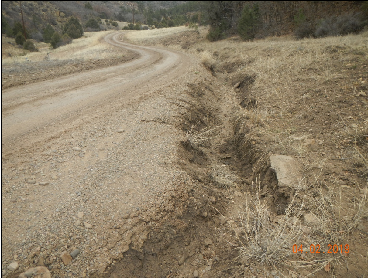
Photo 1. There is an erosion channel that developed at the southeast side of the location along the access road.
