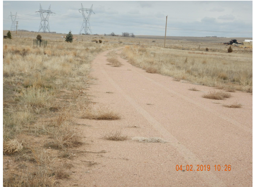
Photo 4. Photo taken of the access road, facing North. See comments under Photo 1.
