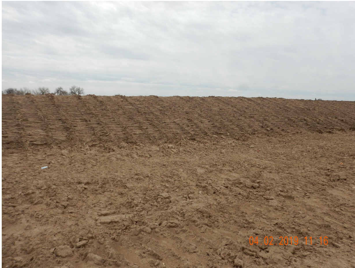
Photo 5. Photo taken from the north-facing topsoil stockpile side on April 2, 2019, facing South. Operator has only stabilized the north-facing side and not the south-facing side.
