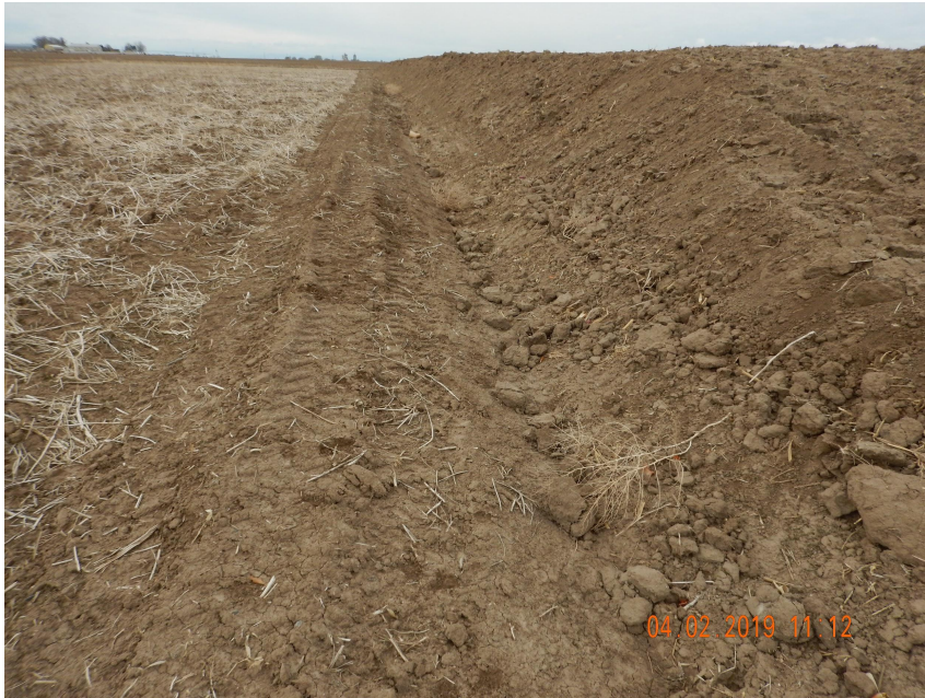
Photo 3. Photo taken from the eastern topsoil stockpile on April 2, 2019, facing West. Operator has failed to stabilize the south-facing topsoil stockpile side since the previous inspection on 3/12/19. Also, leaving the stockpile steep like this would make it difficult to manage weed establishment.
