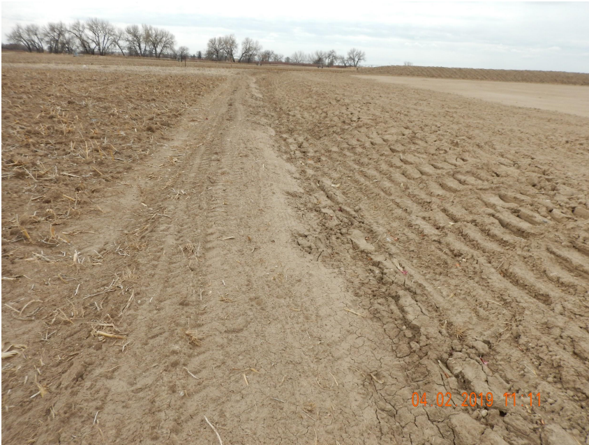
Photo 1. Photo taken from the eastern location, facing South. Photo illustrates a ditch and berm BMP, and the fill slope has been tracked.
