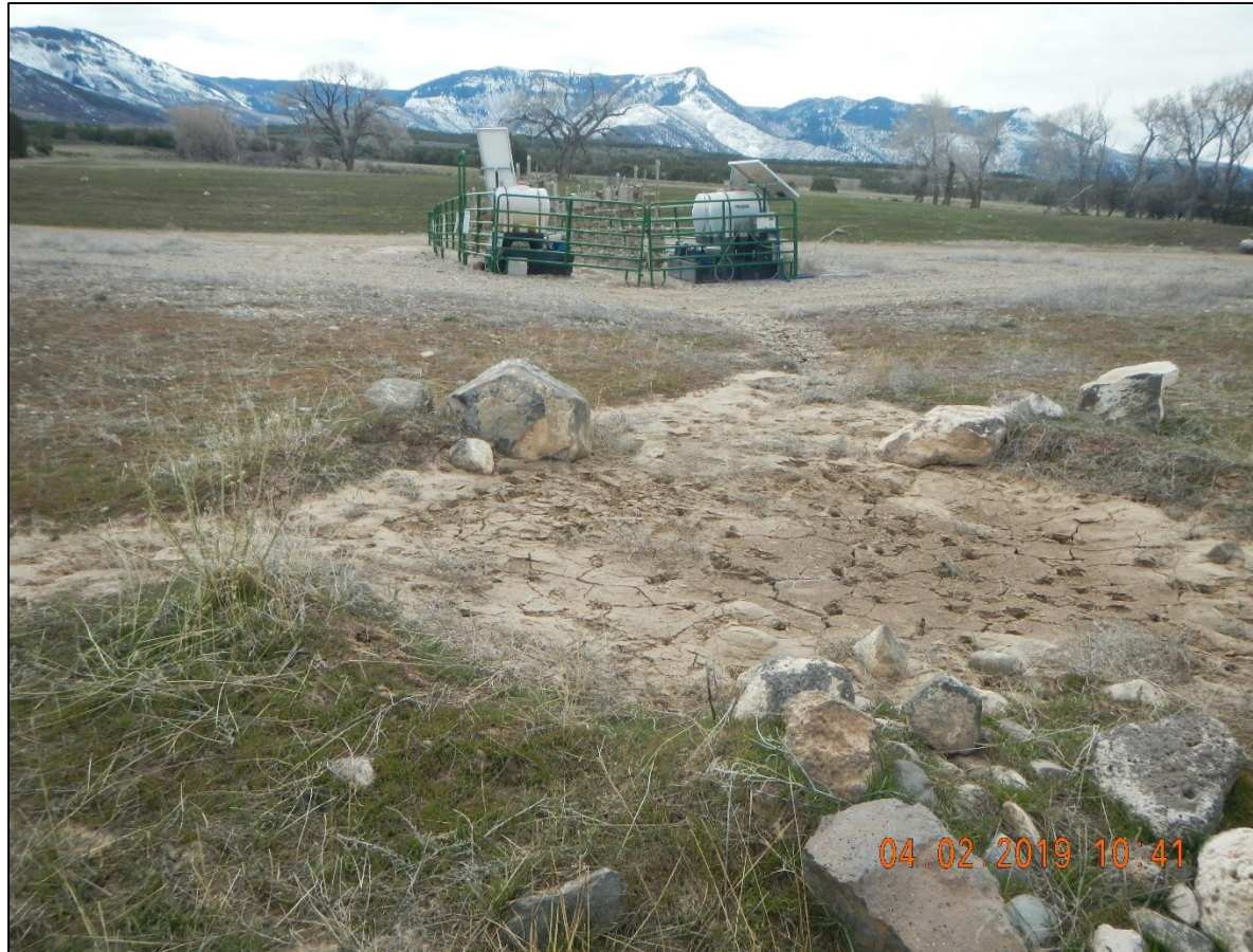
Sediment build up in checkdam.
