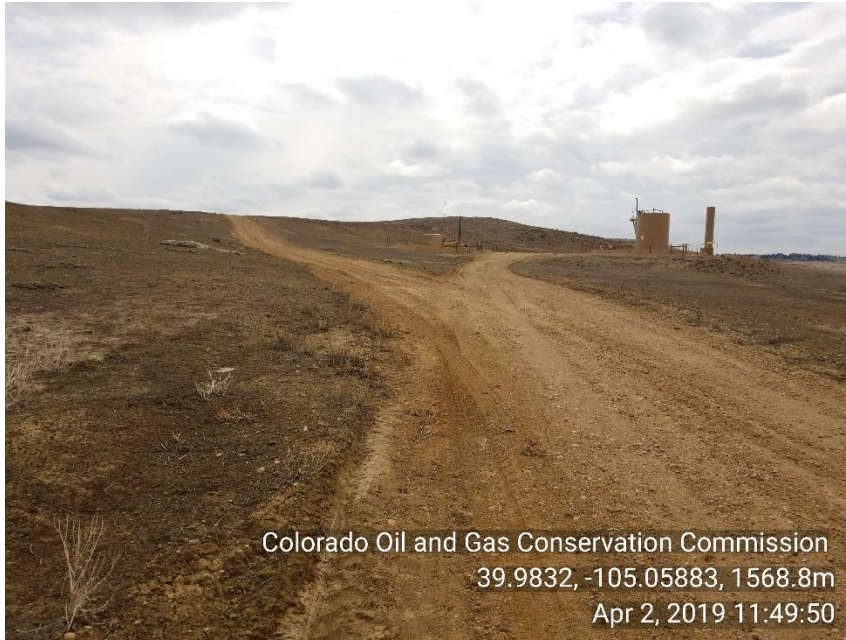
Photo 7 Repairs to road
