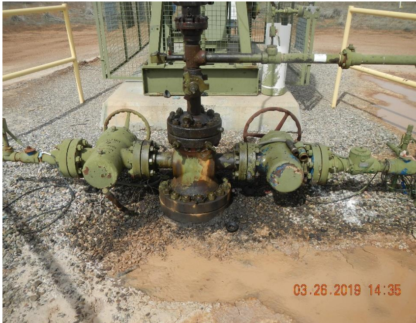
Schuyler 34-9 #30-2 well head is stained and wet. Stained gravel surrounding well head.
