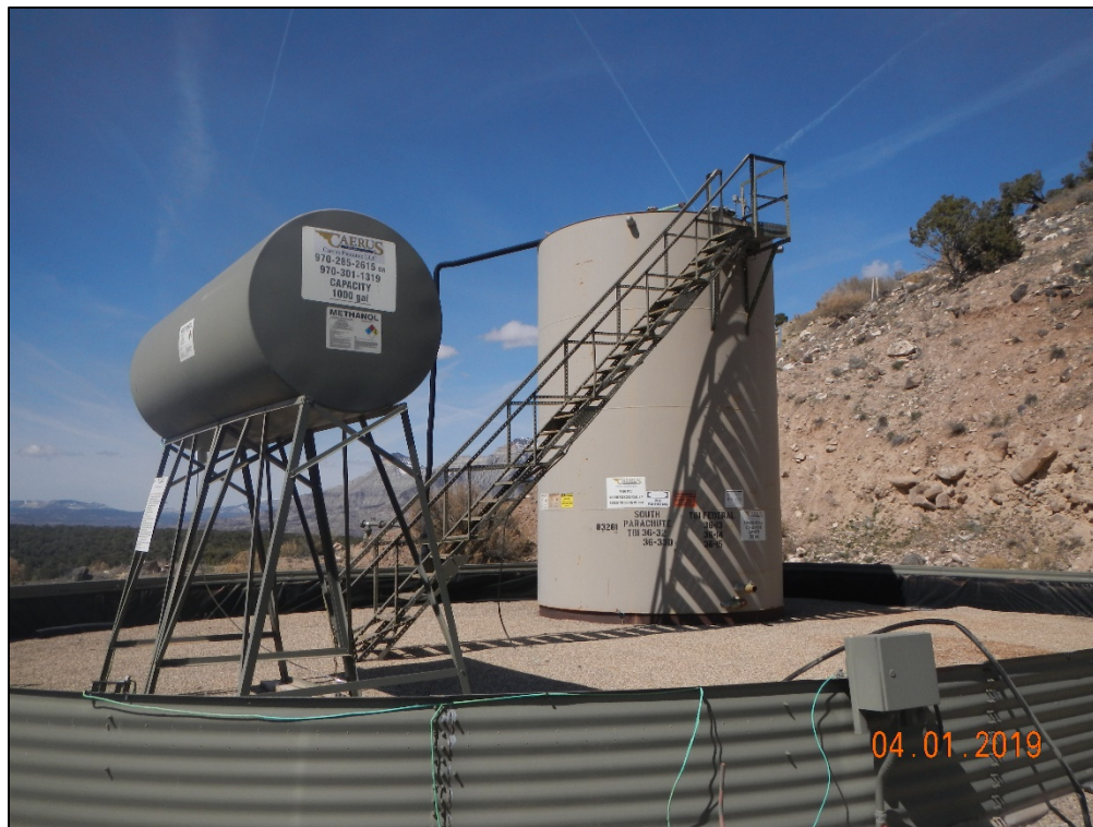
Photo of Tank Battery.
