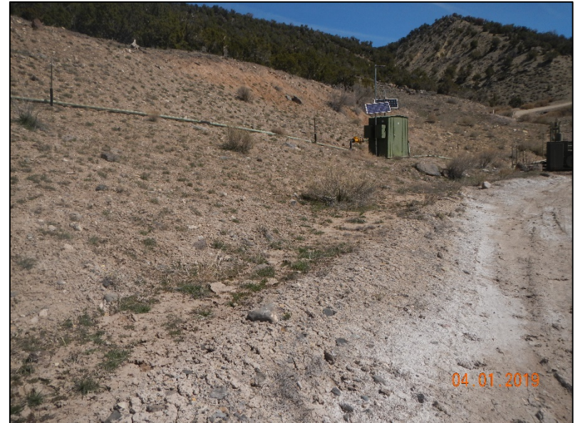
Erosion is evident along unsterilized slope at the north side of location .
