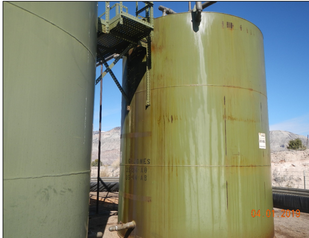
Oily substance staining outside of tank
