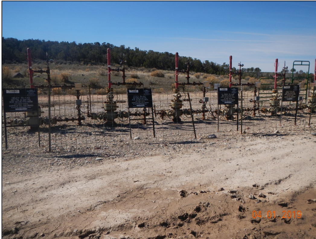
Wellhead signs heavy rutting, loss of compaction
