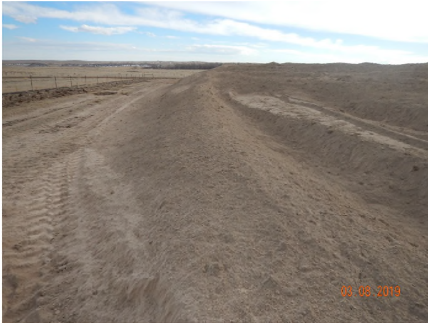
COGCC Photo 11. Photo taken from the east end of the location, facing south. Photo shows unstabilized soils on location at risk to erosion degradation.
