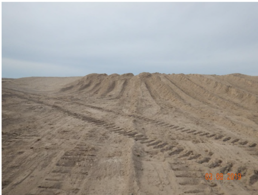
COGCC Photo 12. Photo taken from the south end of the location, facing north. Photo shows unstabilized soils on location at the risk to erosion degradation.
