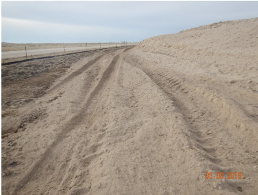
COGCC Photo 13. Photo taken from the south end of the location, facing west. Photo shows unstabilized soils on location at risk to erosion degradation.
