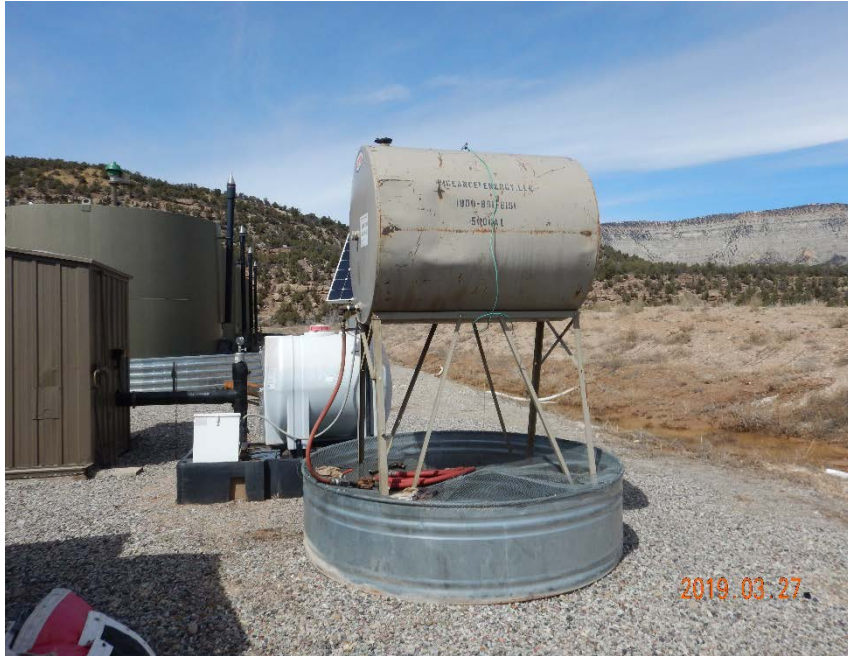
Photo #13 – Day tanks located on NE side of pad.
