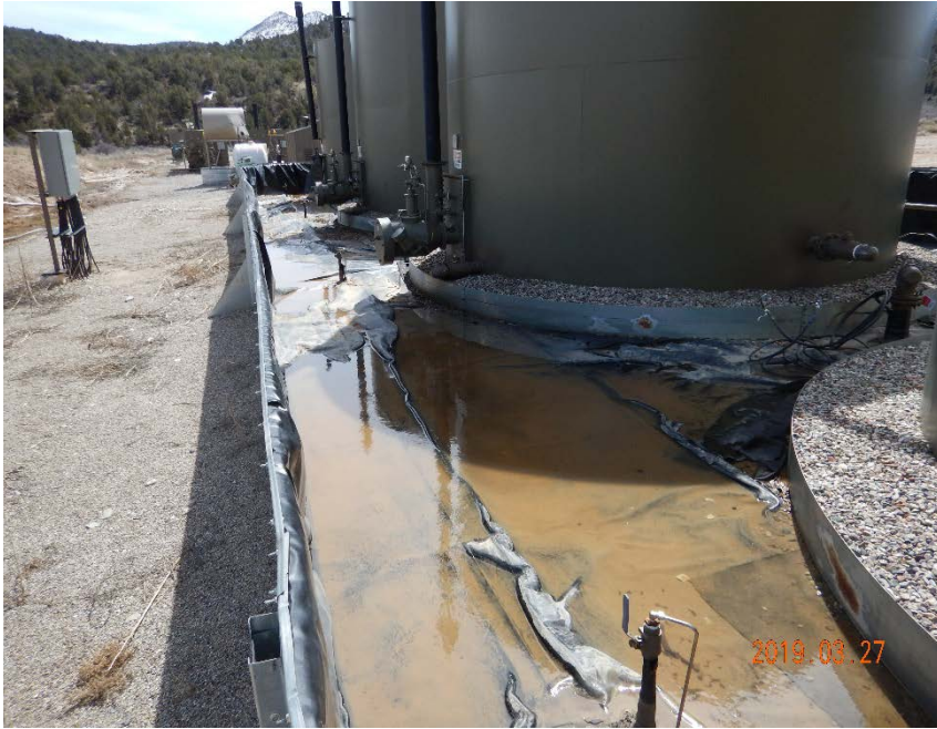
Photo #3 – Flowline risers remaining inside of secondary containment for tank battery (northeast side).
