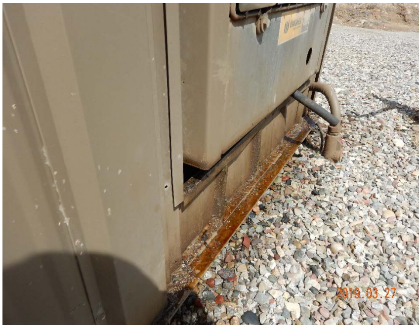
Photo #11 – Lube oil and oil-stained gravel on south side of shed.
