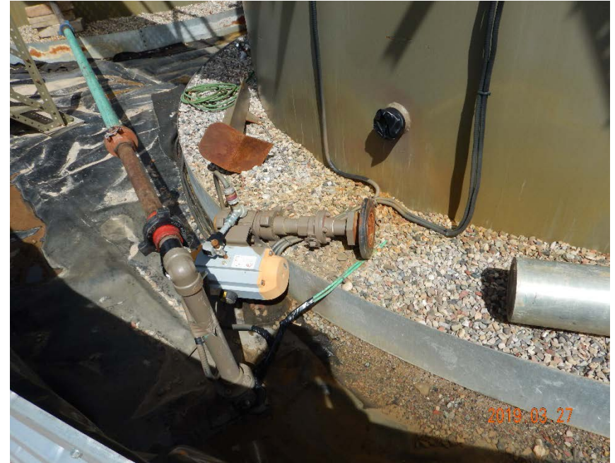
Photo #2 – South produced water tank was disconnected on inspection date.
