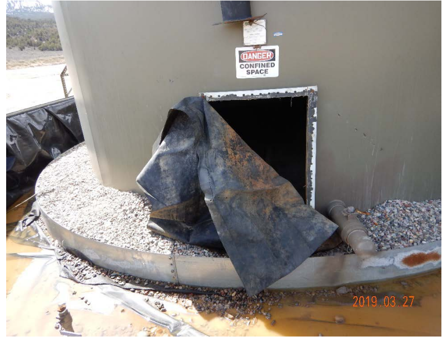
Photo #4 – Open access panel on east side of south produced water AST.
