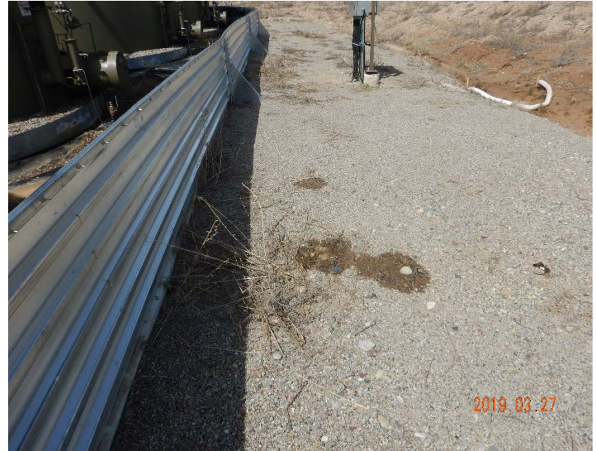
Photo #6 – Localized, stained soil outside of tank battery secondary containment (northeast side).
