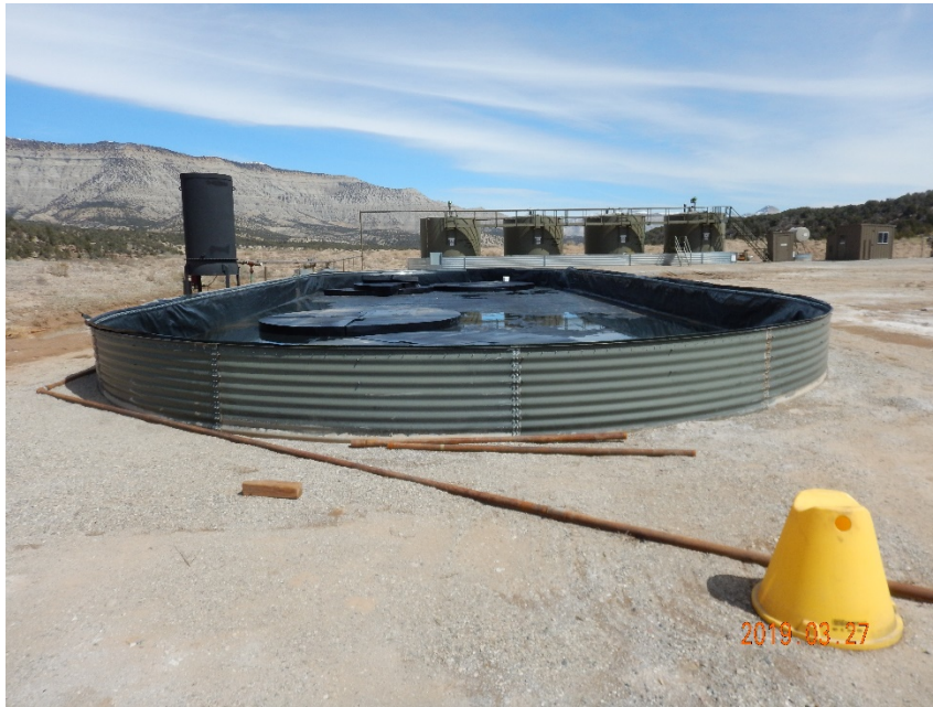
Photo #7 – Tank battery under construction on northwest side of pad. Note proximity of tank battery containment to ECD on left side of photo.
