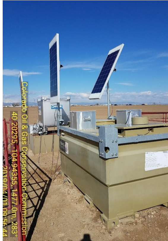
Photo 5 Corrosion Inhibitor and Methanol Tanks with Secondary Containment
