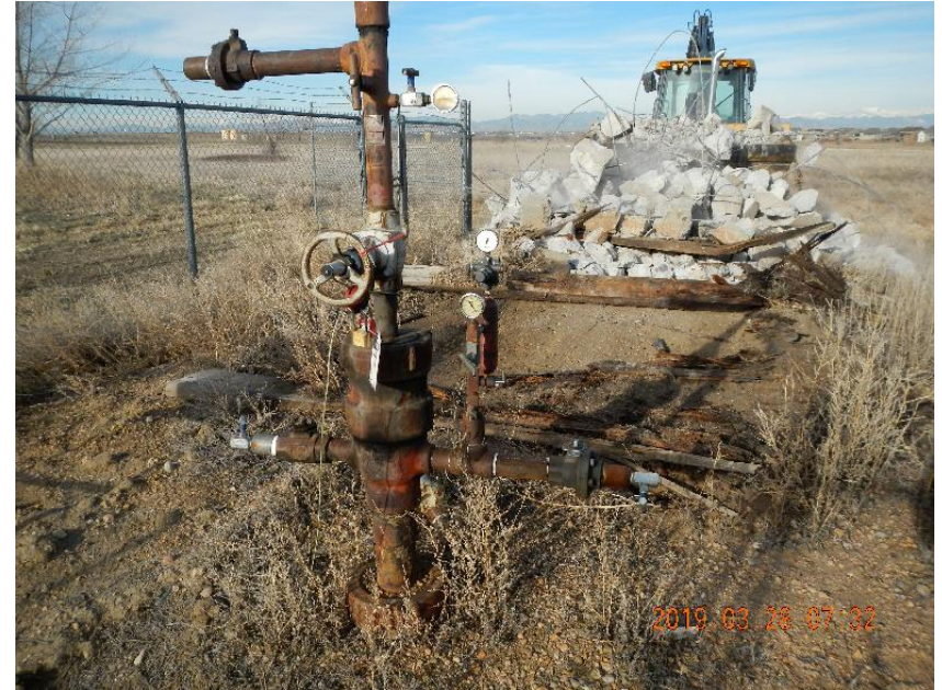
Photo 2: Loading concrete from pumping unit base.
