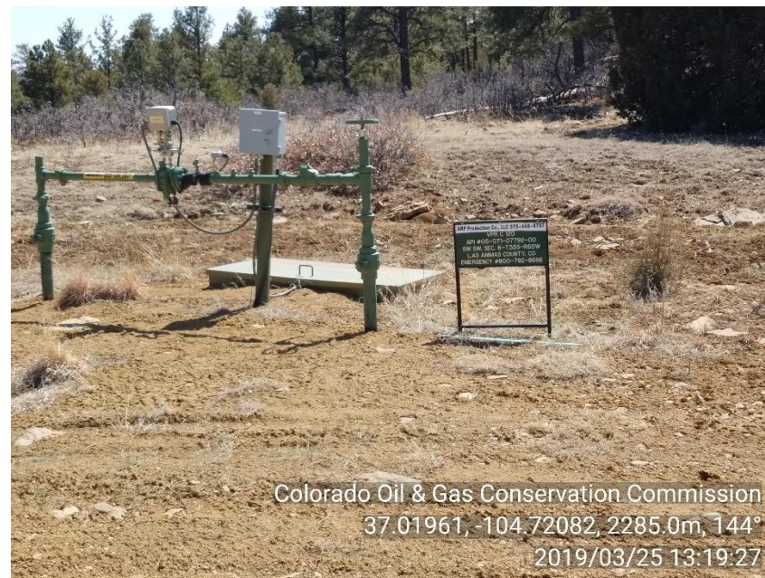
PHOTO 2: LOCATION SIGN/ METER RUN
