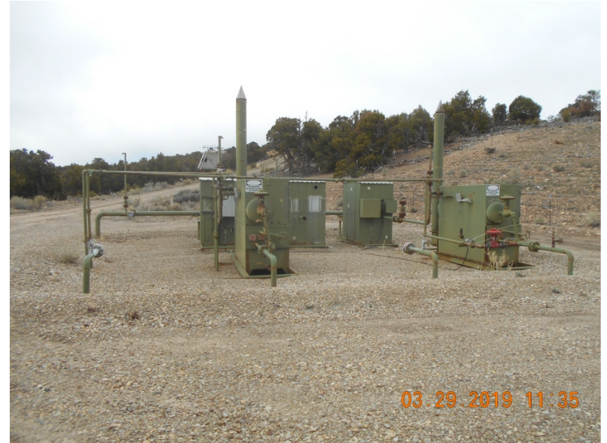
Separators and meter housing.
