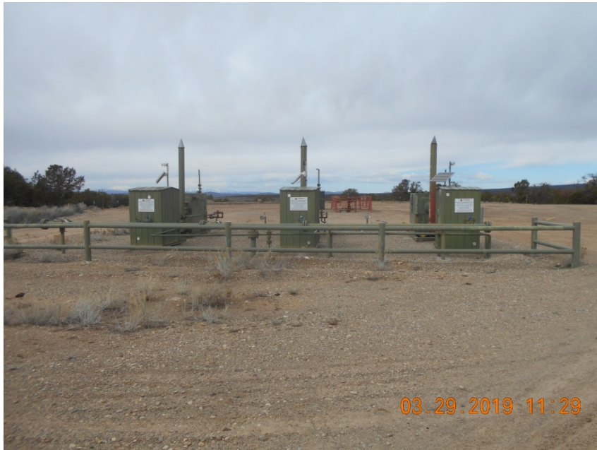
Meter housings w/ signs and pipe barricade
