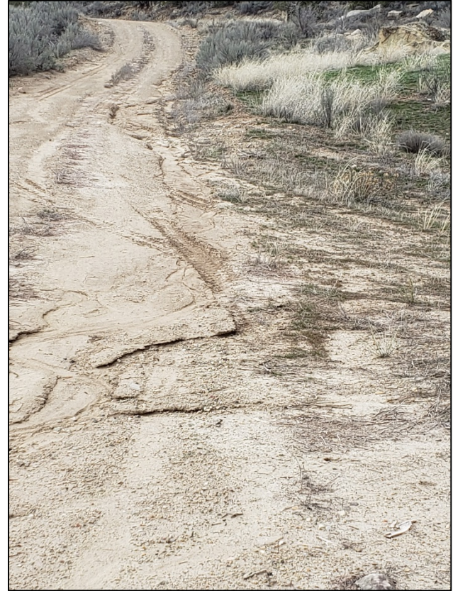
Erosion from upper location coming down access road and running onto location
