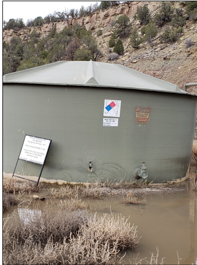
Photo of Tank Battery. Berm has debris around it and fluid in containment
