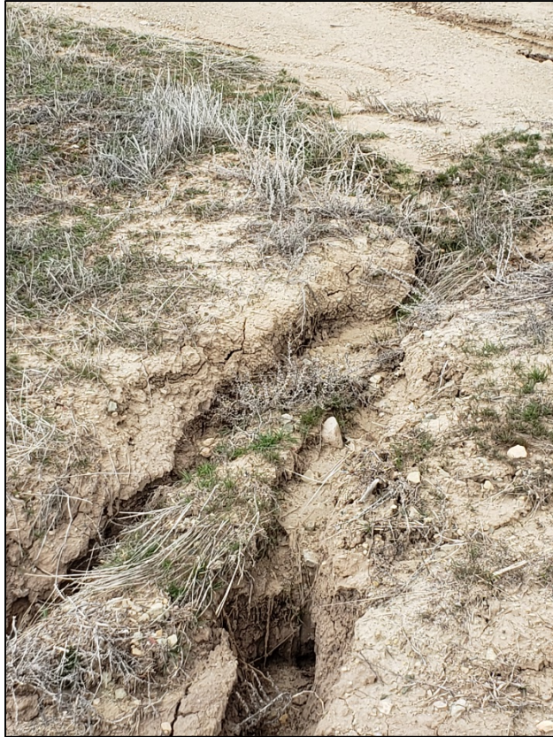
Erosion from location going down the access road
