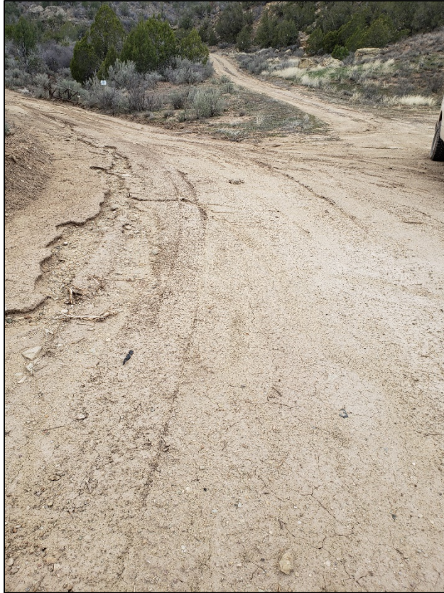
Erosion leaving location from BMP not being maintained
