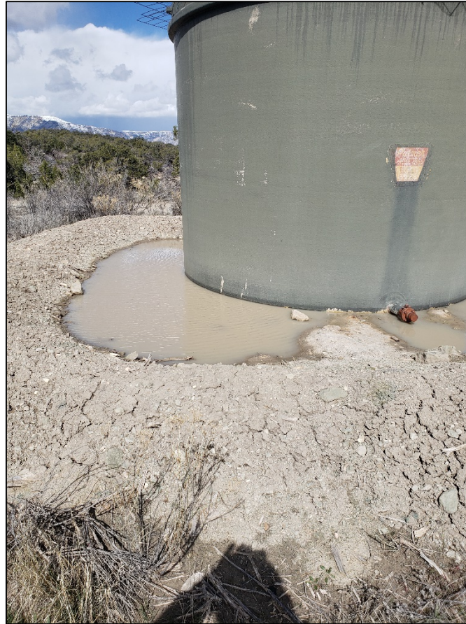
Faded label on tank and fluid in tank battery containment
