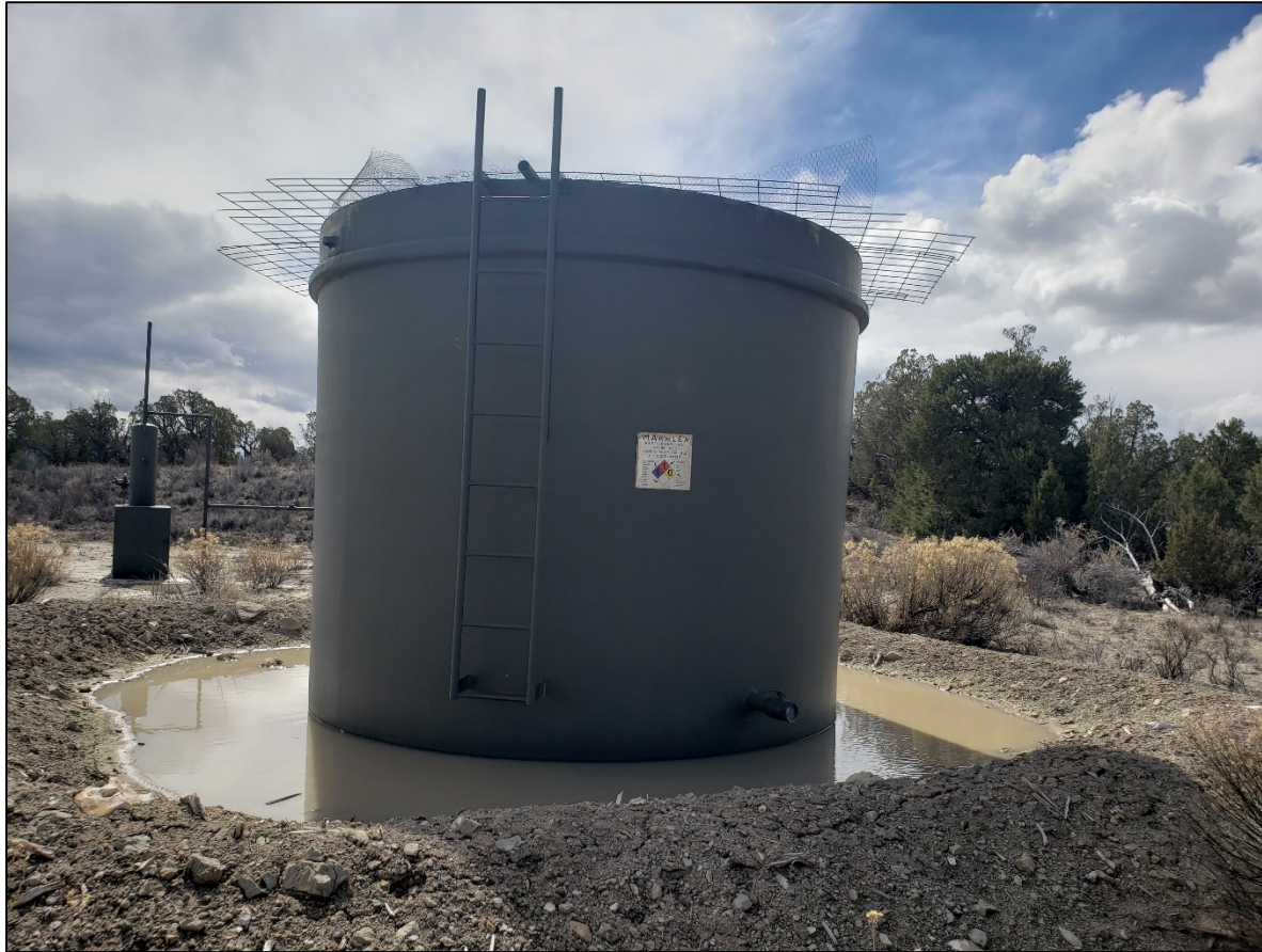
Photo of Tank Battery. Berm full of fluid
