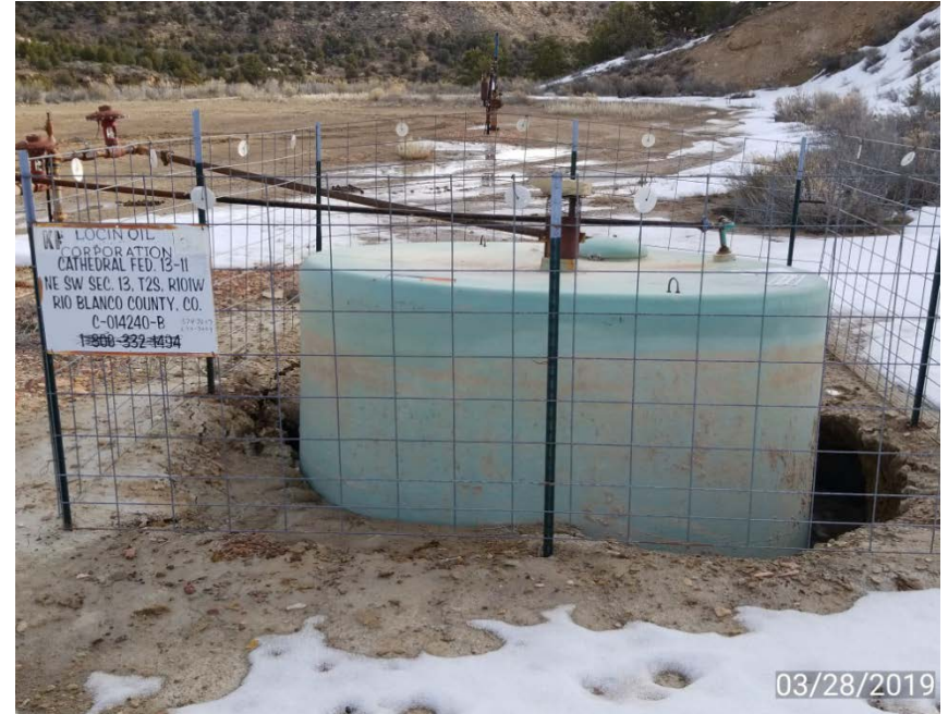
Photo 2. Tank without berm.
