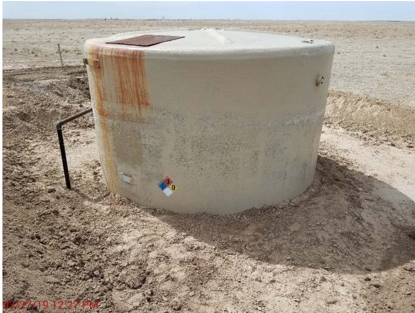
Photo 7 – New produced water partially buried vessel. No contents label.
