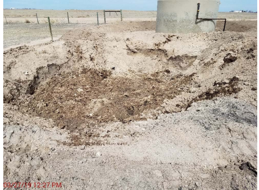
Photo 10 – Produced water pit from south berm. Oily waste in pit.
