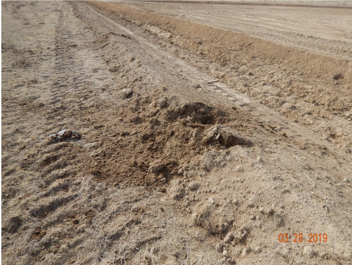
Photo 5: Photo taken from the ditch/berm on the east end of the location. Photo shows operator has installed a ditch/berm BMP along perimeter of the location. BMP does not appear to have been constructed in accordance with good engineering practices; BMPs have not been sufficiently compacted, remains unconsolidated materials and a potential source for sediment laden stormwater discharge.
