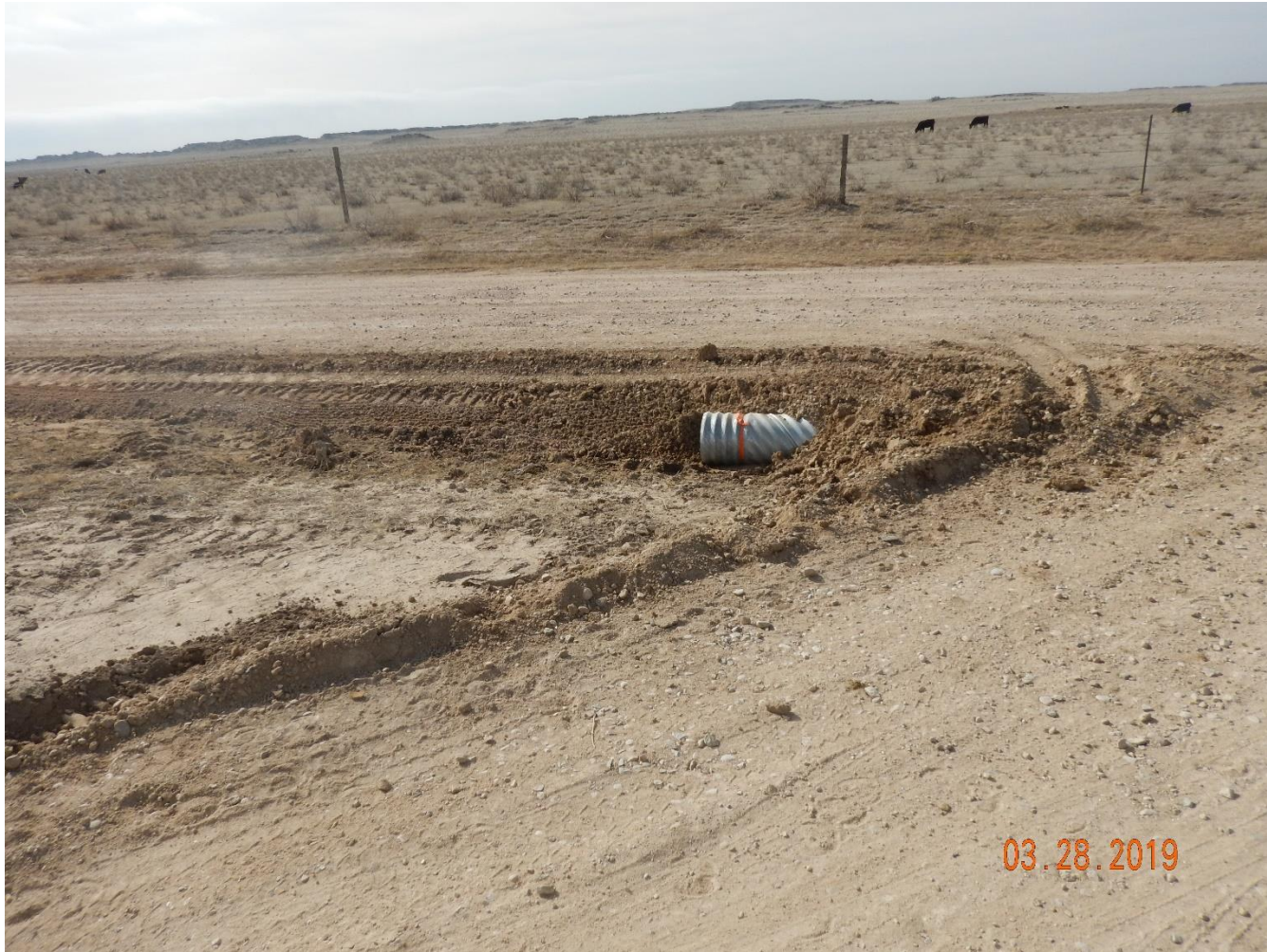
Photo 8: Photo shows culvert installed and access road.
