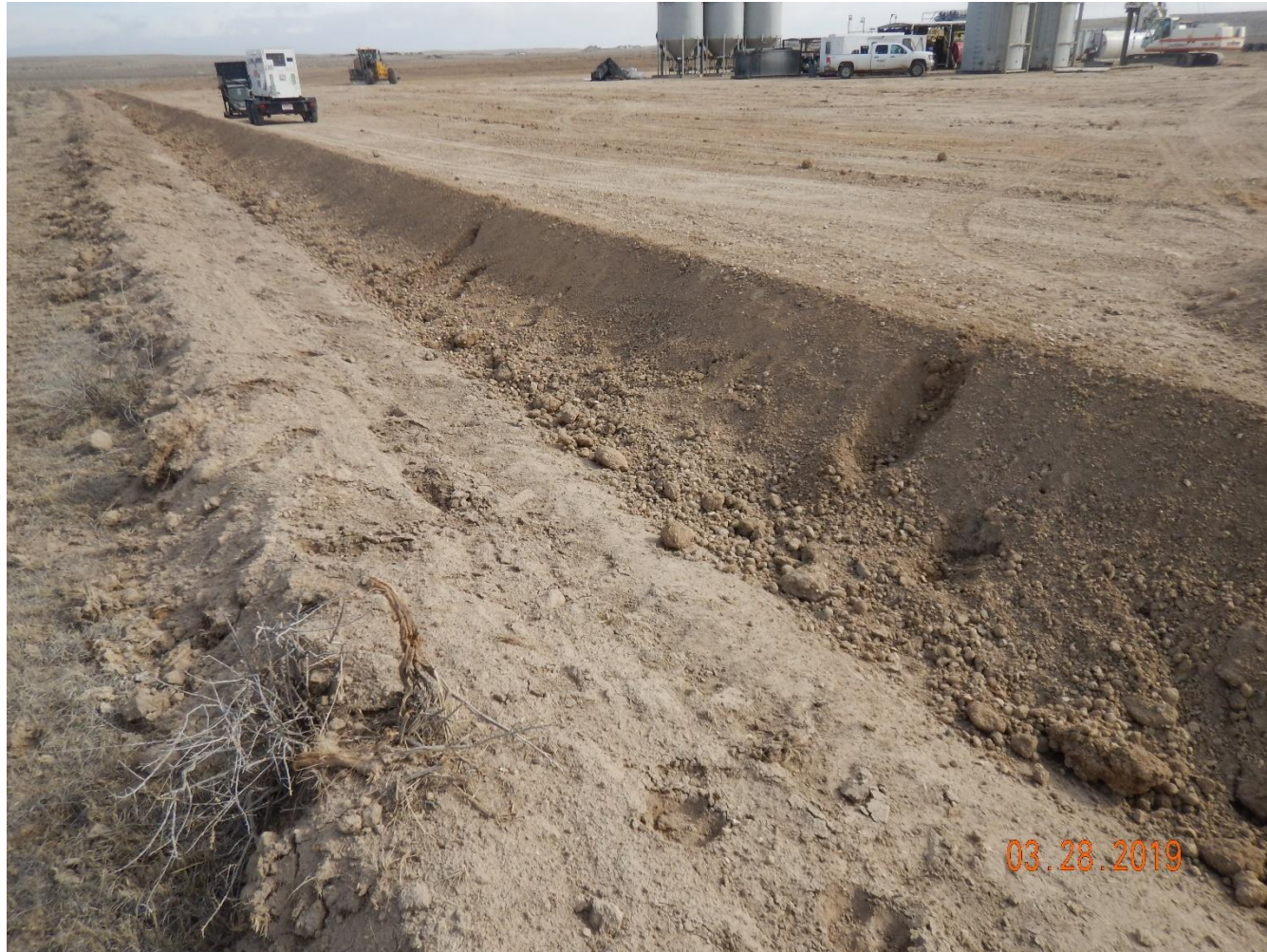
Photo 3: Photo taken from the ditch/berm on the west end of the location, facing northeast. Photo shows operator has installed a ditch/berm BMP along perimeter of the location. BMP does not appear to have been constructed in accordance with good engineering practices; BMPs have not been sufficiently compacted, remains unconsolidated materials and a potential source for sediment laden stormwater discharge.
