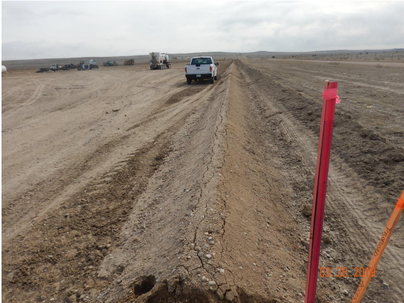
Photo 1: Photo taken from the southwest corner of the location, facing east. Photo shows operator has installed a ditch/berm BMP along perimeter of the location. BMP does not appear to have been constructed in accordance with good engineering practices; BMPs have not been sufficiently compacted, remains unconsolidated materials and a potential source for sediment laden stormwater discharge.
