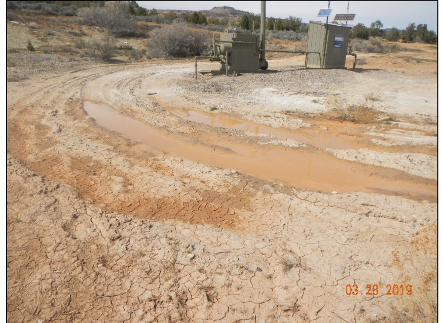
Rutting on location , no compaction or gravel in all areas
