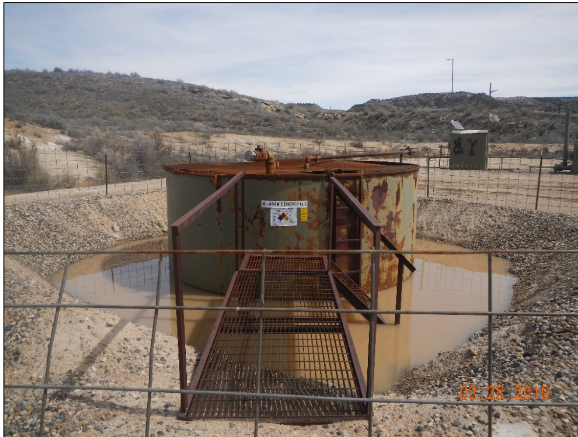
Photo of Tank Battery. Rust on tank
