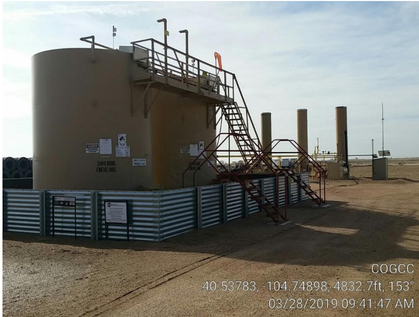
Photo 3 – Tank Battery
