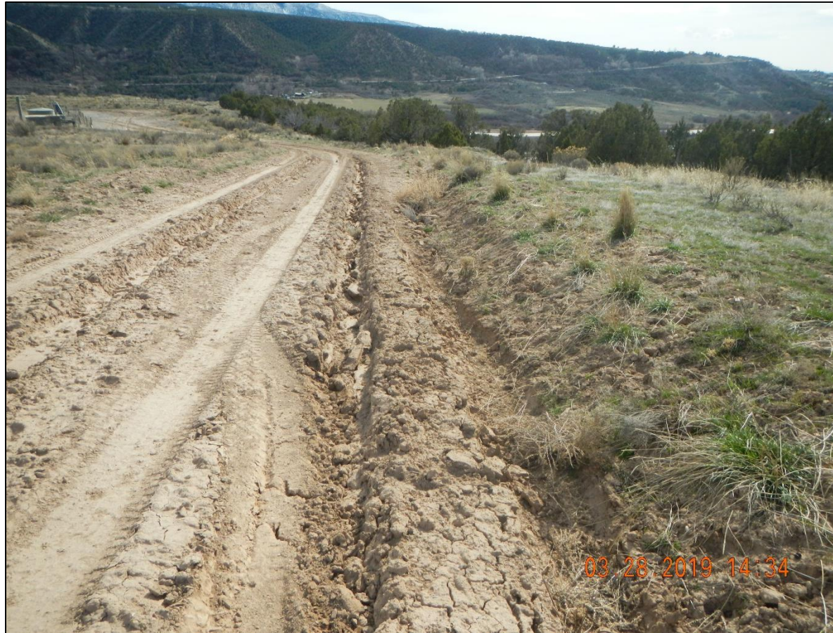
Rutted road and ditch in disrepair.
