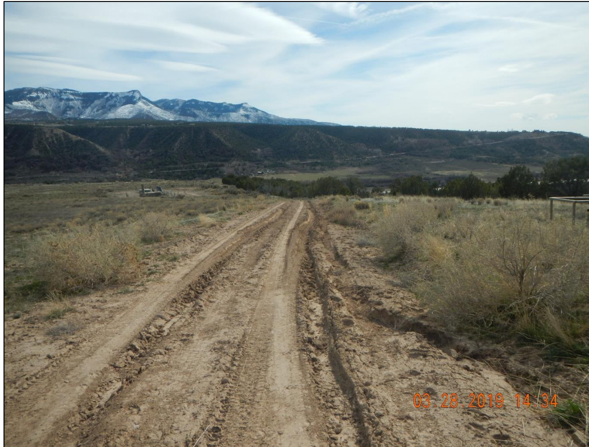
Rutted road and ditch in disrepair.
