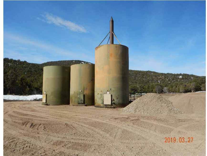
Photo #2 – Unused production tanks had been relocated from tank battery area to center of pad prior to inspection date.
