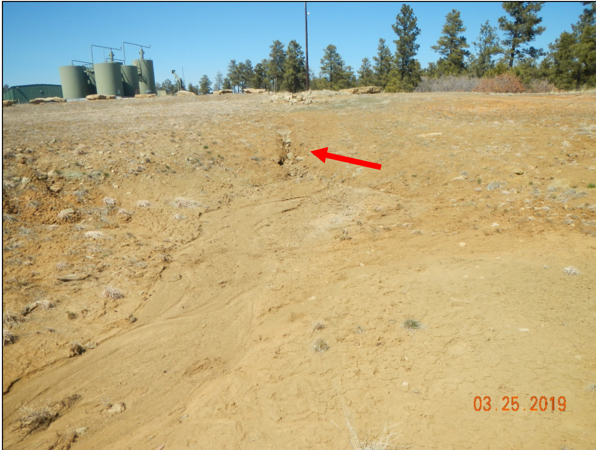
Photo 4. Facing west at the north side of the location. There is signs of erosion in this area.
