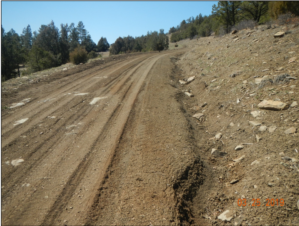
Photo 1. Facing southwest along the access road. No BMP's are installed to prevent erosion along the side of the access road.
