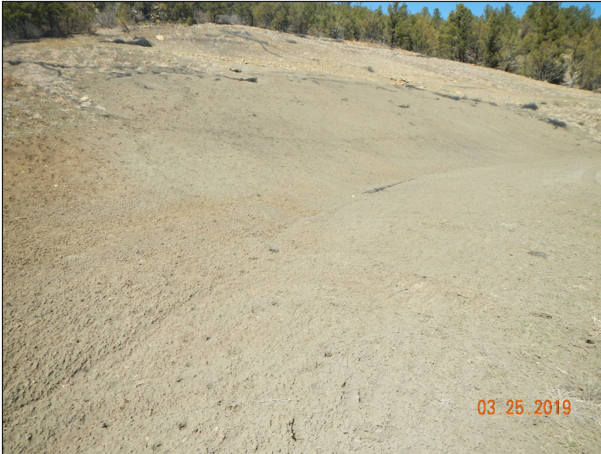
Photo 2. The cut slope is bare of vegetation and susceptible to erosion.
