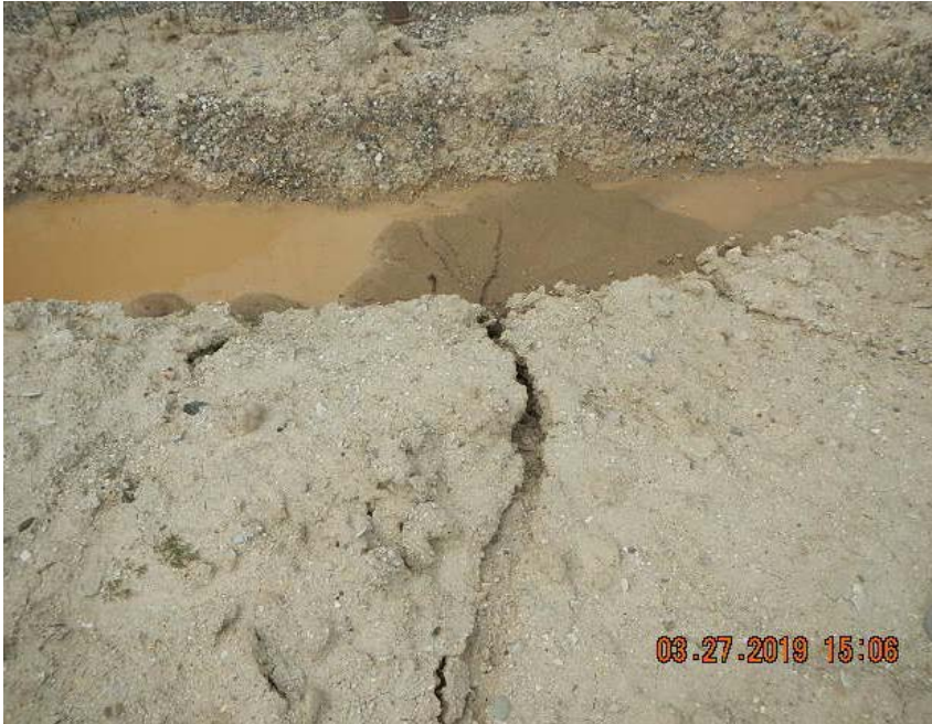
Erosion is evident along unsterilized slope at the east side of location .
