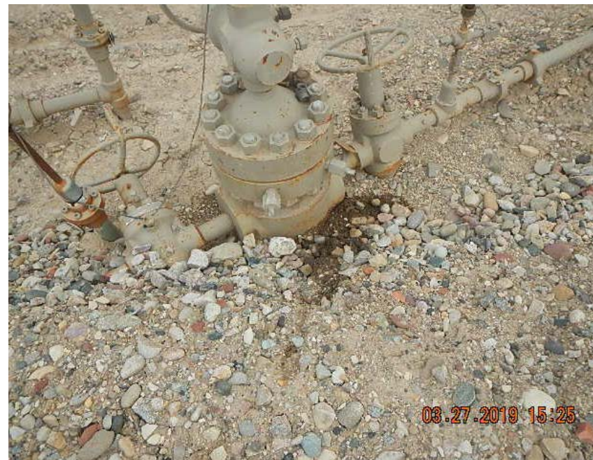
Staining around well head
