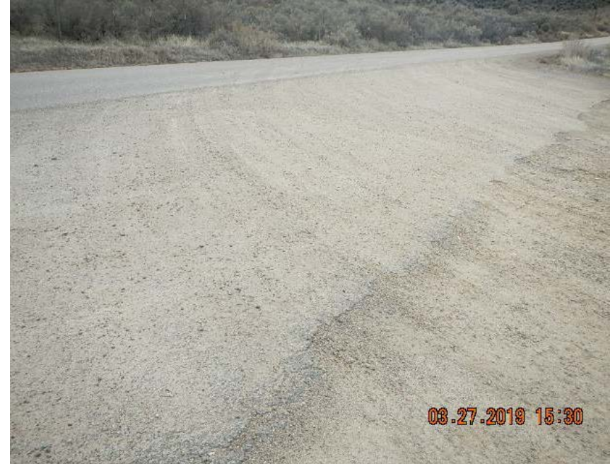
Tracking onto CR 320 from location 334745. No tracking BMP in place.
