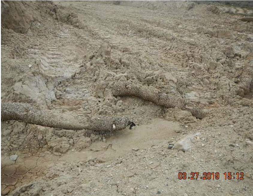
BMP damaged and not maintained at the NW corner of location.
