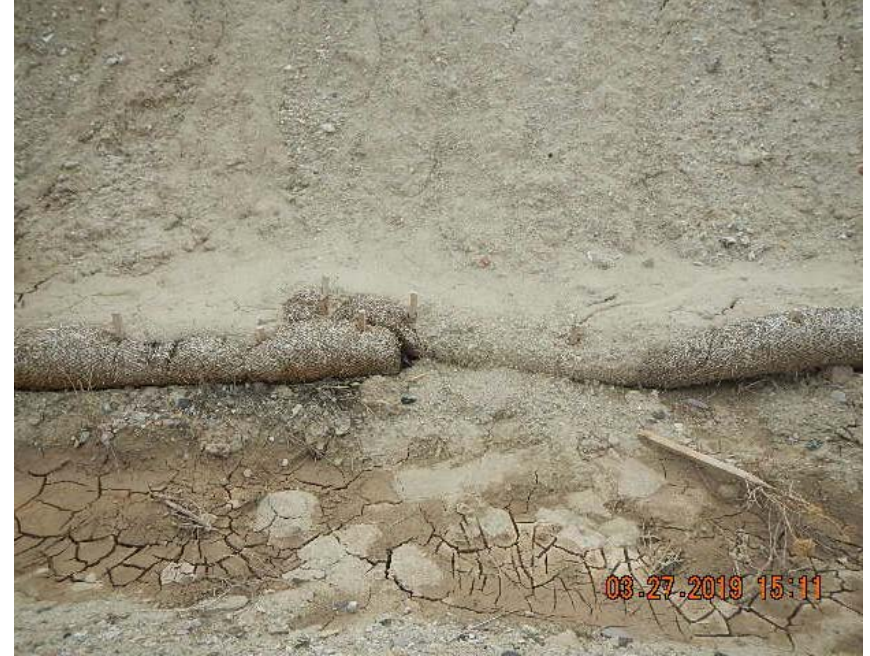
BMP not maintained on NE edge of location.
