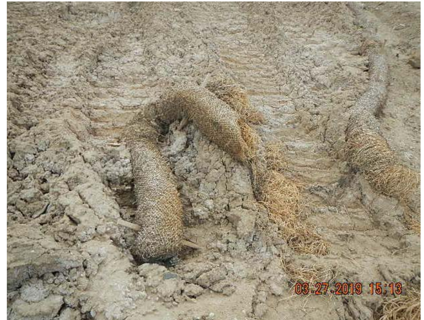
BMP damaged and not maintained at the NW corner of location.
