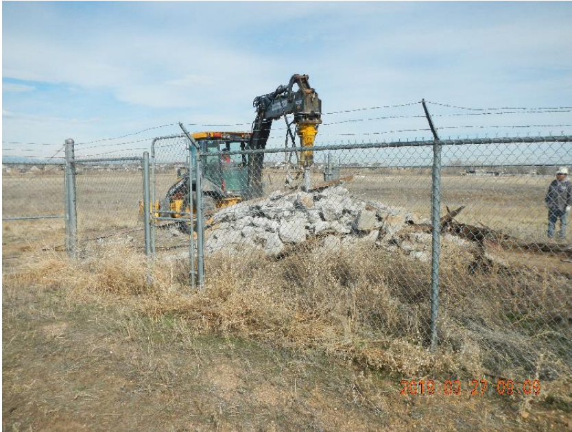
Photo 3: Additional view of braking up base.
