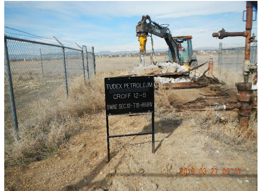
Photo 2: Breaking up concrete pumping unit base.
