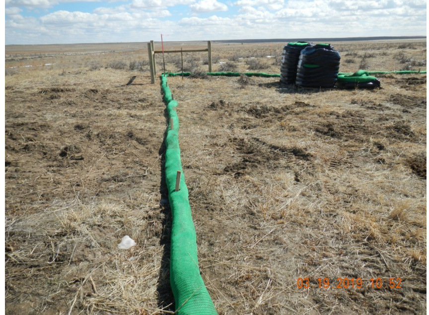
Photo 2. Photo taken from the northern perimeter of the location, facing East. Photo illustrates a filterxx BMP that has been installed around the perimeter of the location prior to the start of construction. BMPs are in proper functioning condition at the time of this inspection.
